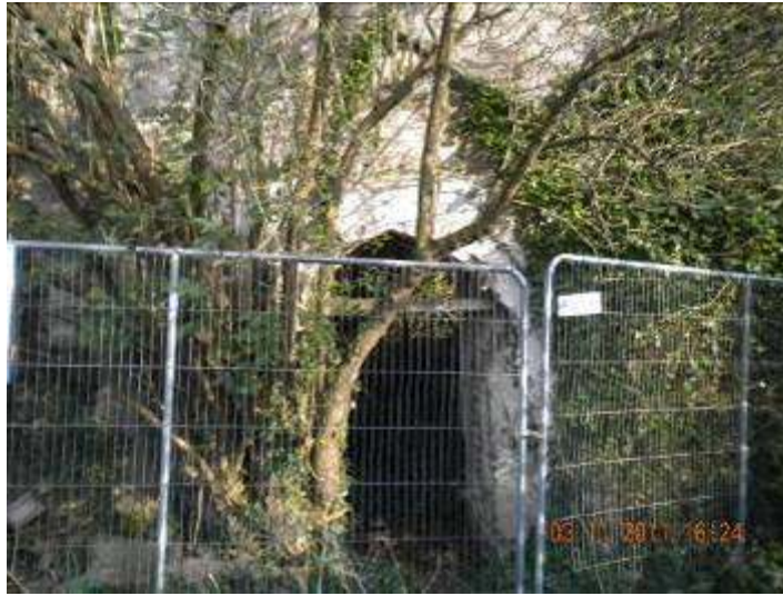
Detail of entrance door on the west side
