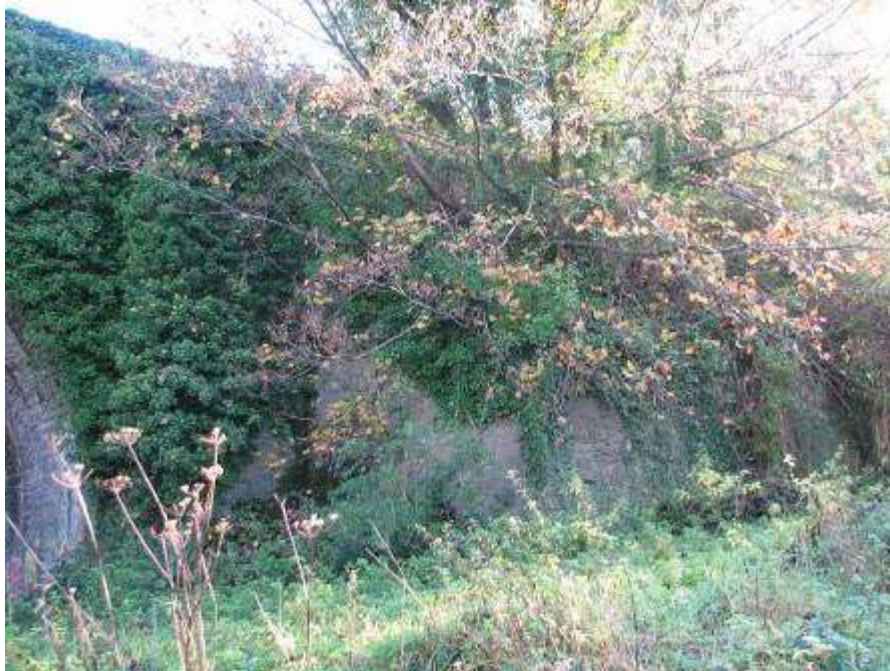
Buttress at south-west corner
