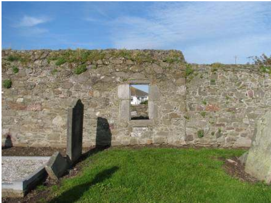
Window on the south wall
