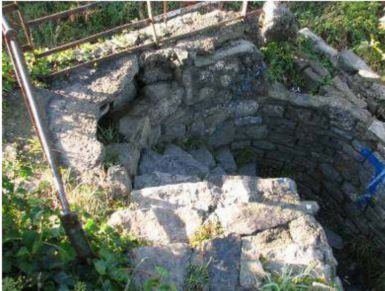
Spiral stair from above
