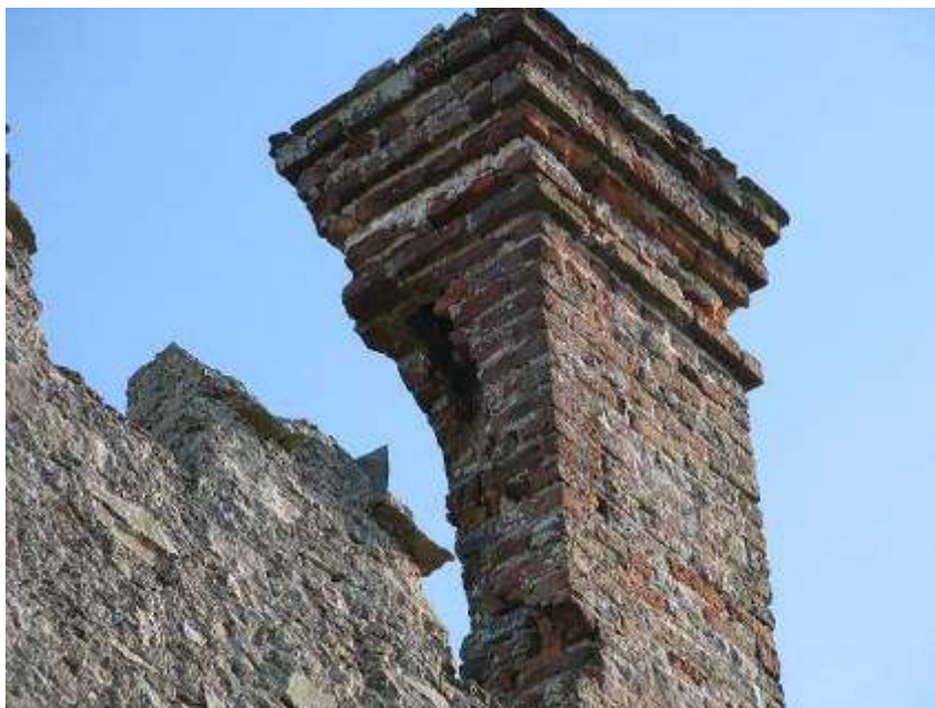
View of the chimney from the north
