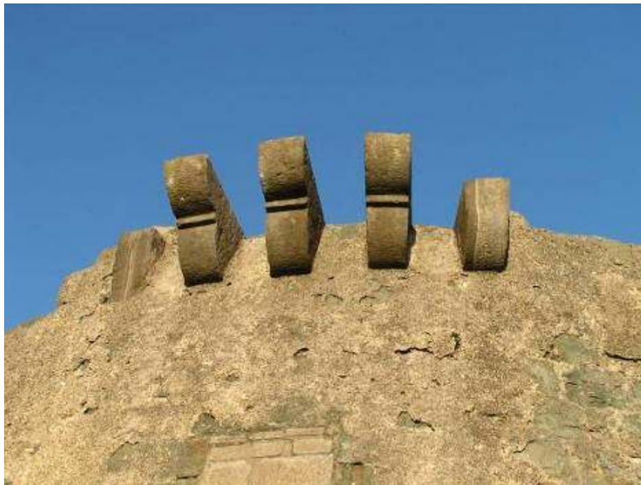
Detail of machicolation brackets
