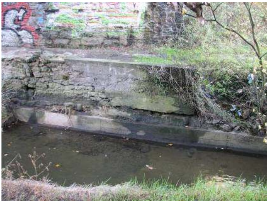
Underpinning at north abutment
