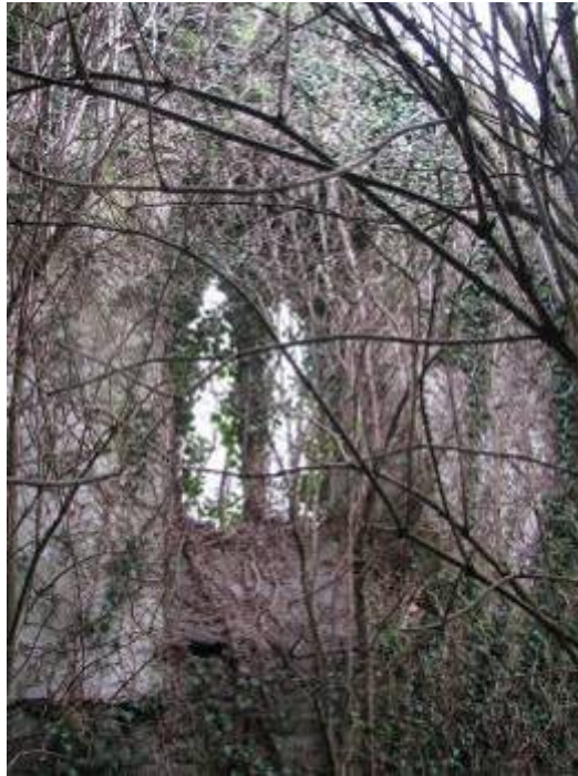
View of the interior – note tree growth
