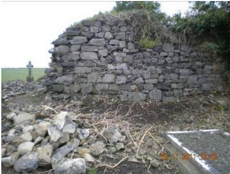
North end of the West wall (West face)
