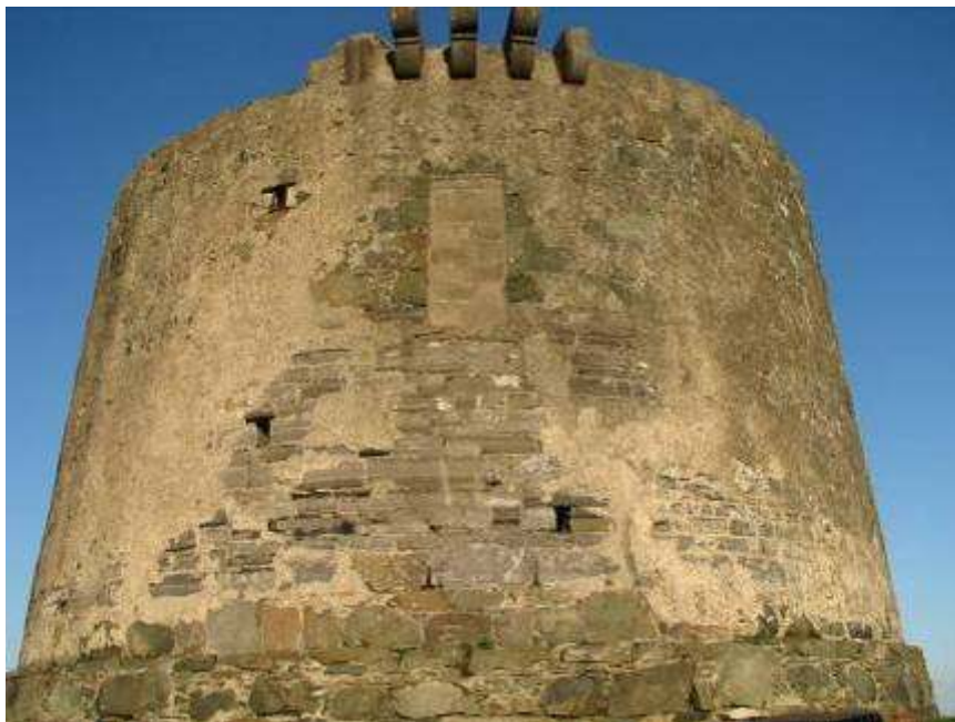
Tower former entrance
