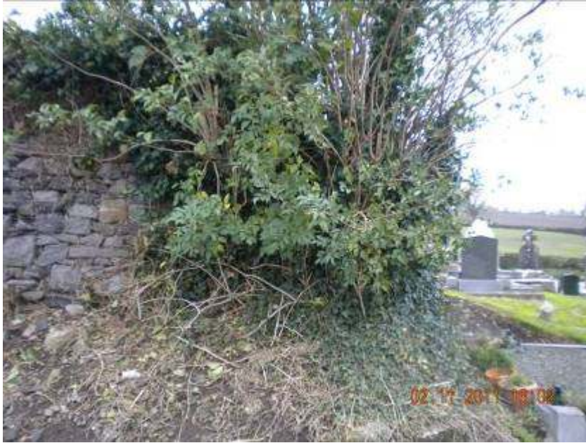
South end of West wall (West face)
