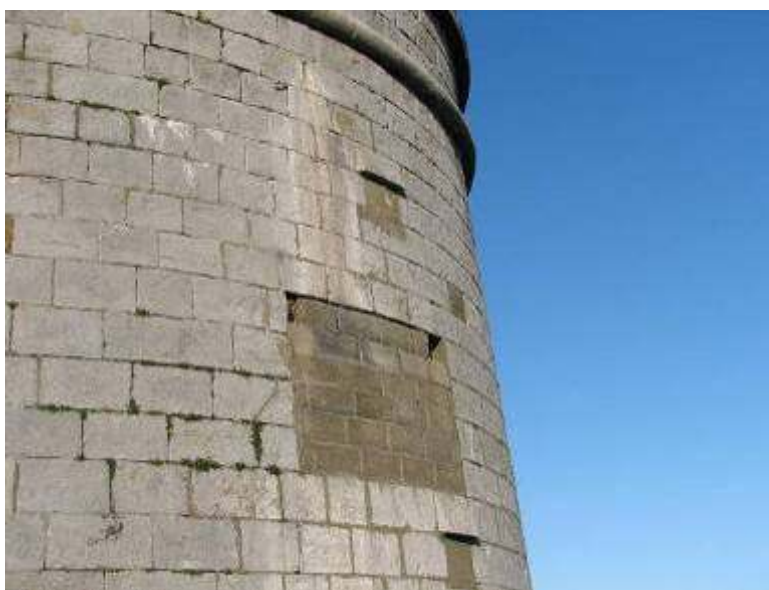
Detail of blocked up former openings
