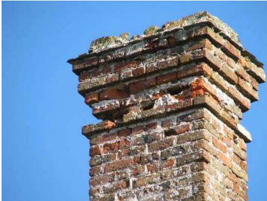
The brick chimney
