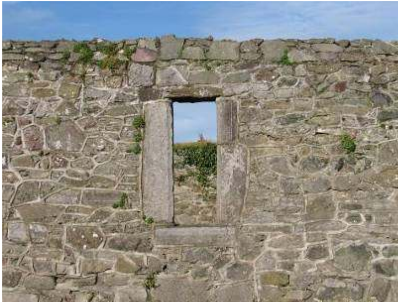
Window opening in the south wall
