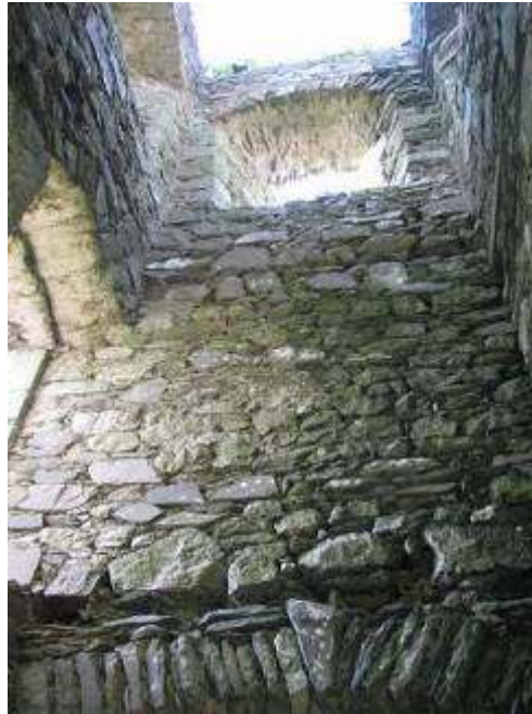
The tower interior west wall
