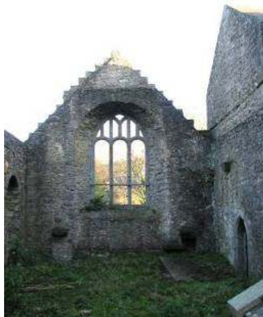
West elevation of east wall
