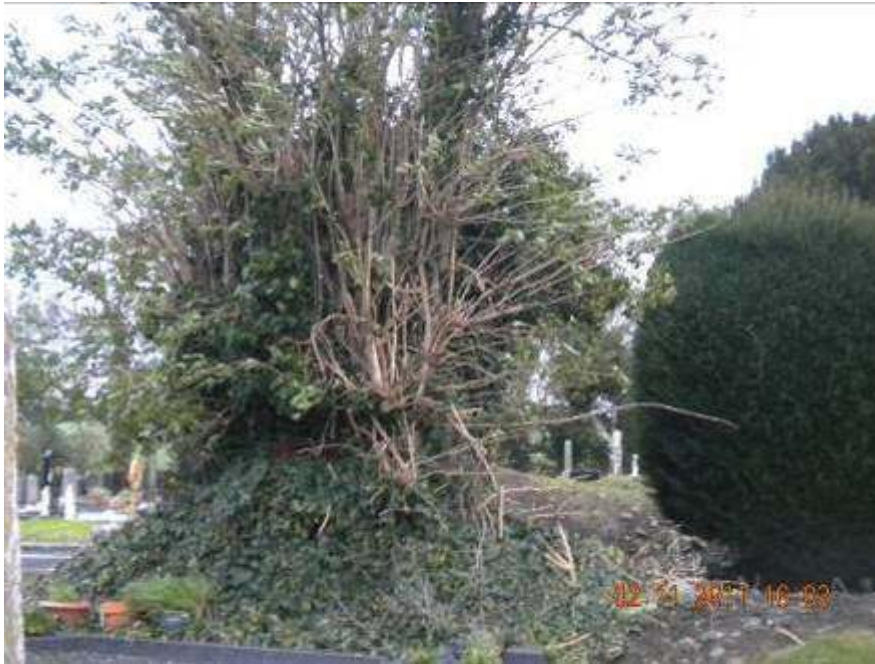
West end of West wall
