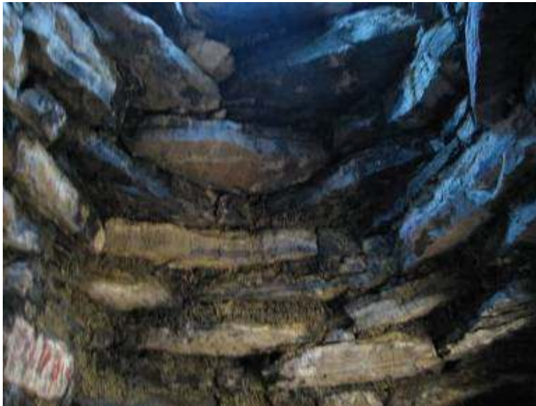
North-east tower – corbelled first floor
