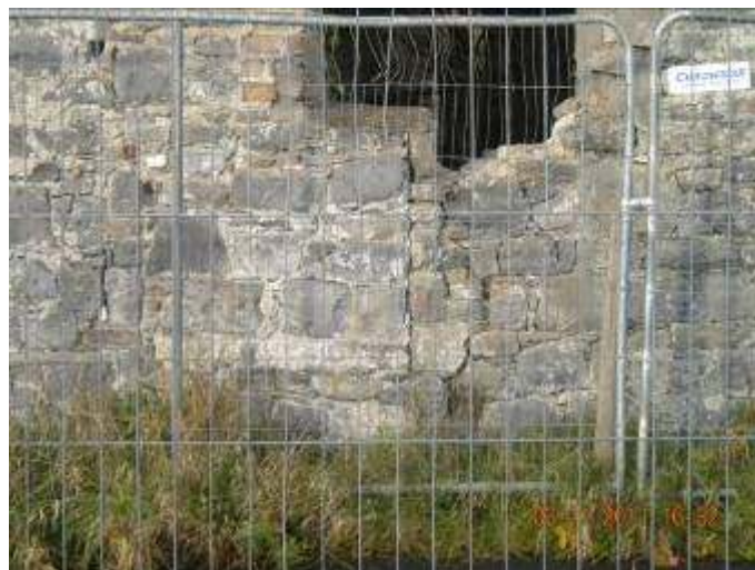
Detail of wall on south side – note construction joint
