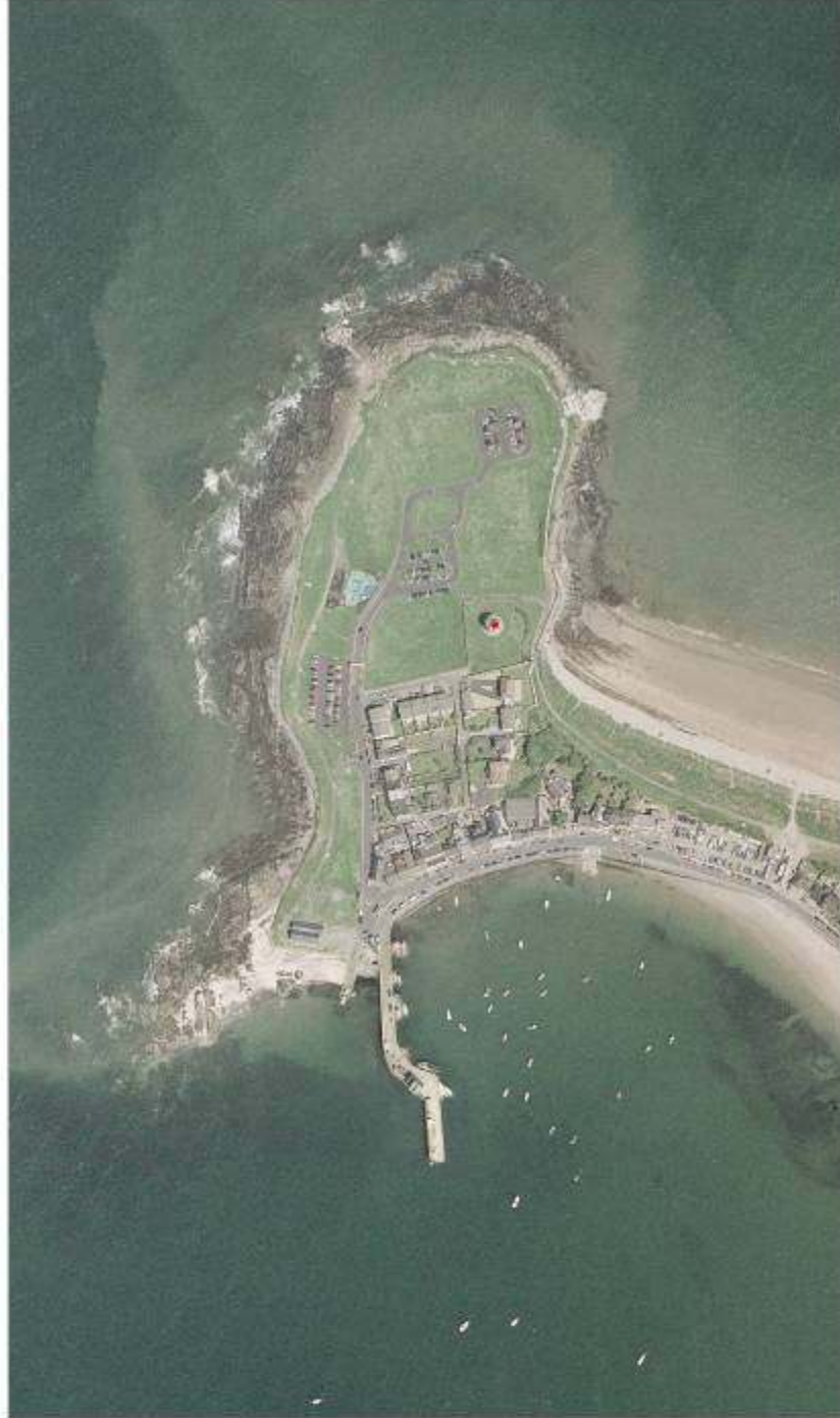
RPS No. 189 Martello Tower, Red Island, Skerries, Co. Dublin
