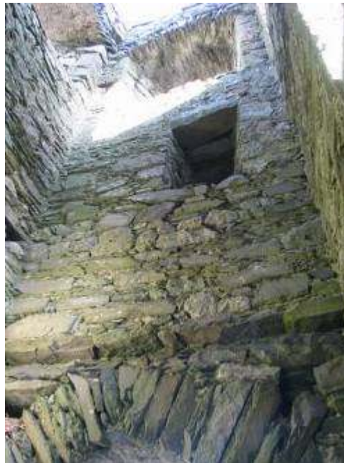
Tower interior east wall
