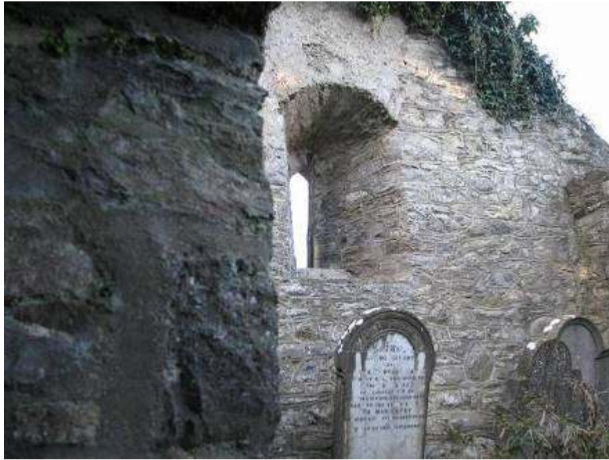
West gable interior (note plaster remnants)
