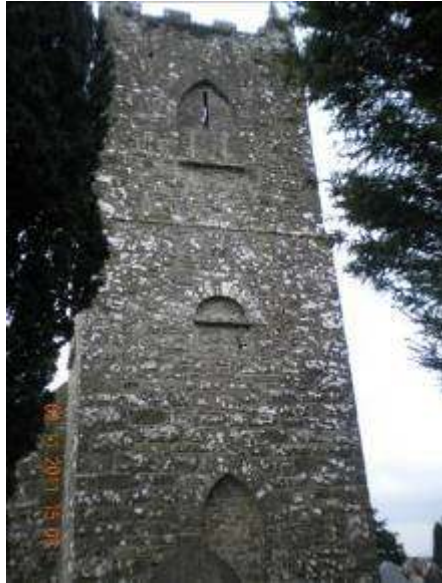
West elevation of the tower
