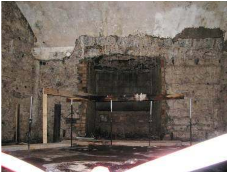
First floor interior – note lime ‘stalactites’
