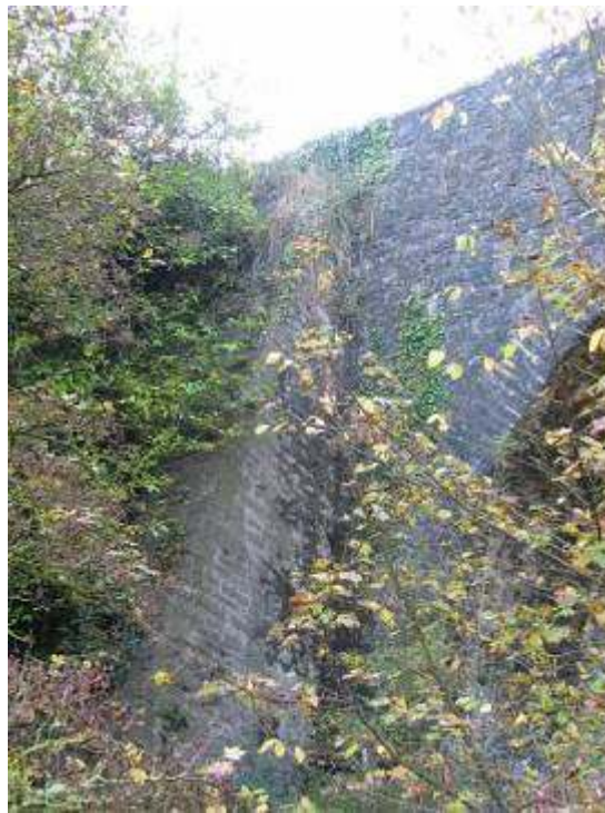
Buttress at south-east corner
