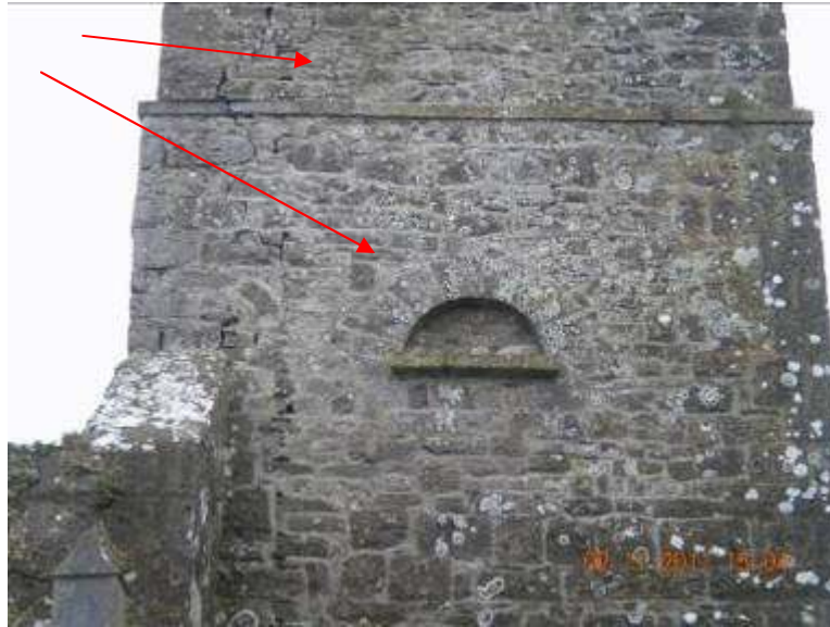
Detail of North tower wall lower level
