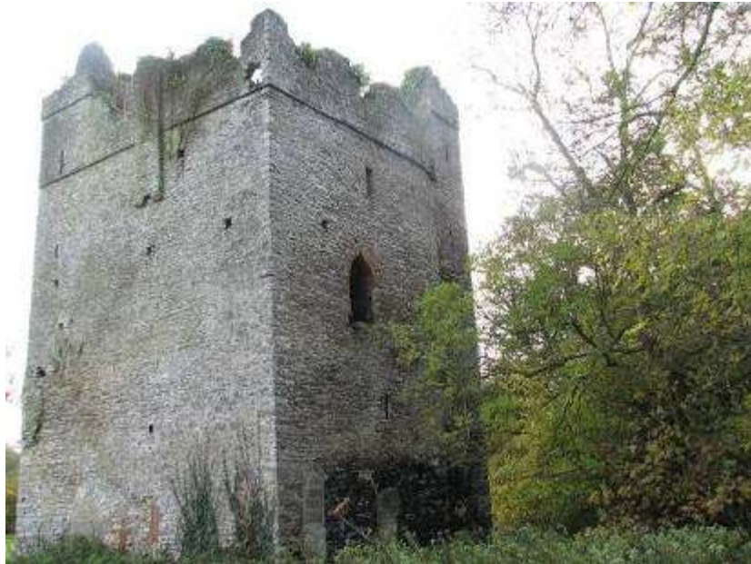
West elevation (from the North-west)
