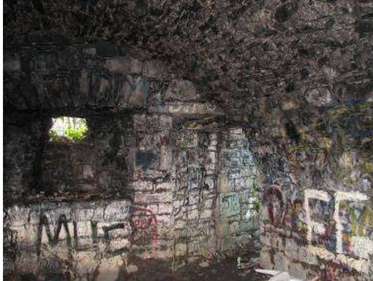
Undercroft – view from entrance
