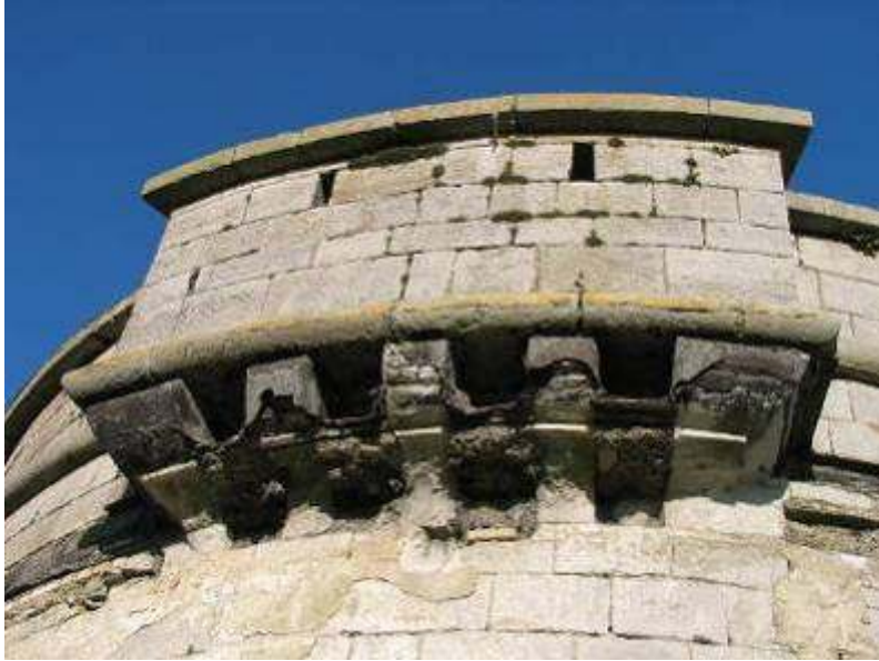
Detail of machicolation with concrete infilling
