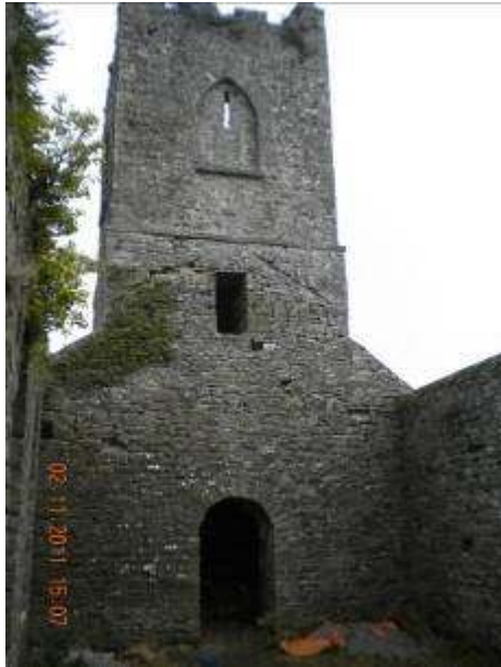
East wall of tower
