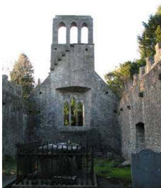
East elevation of west wall
