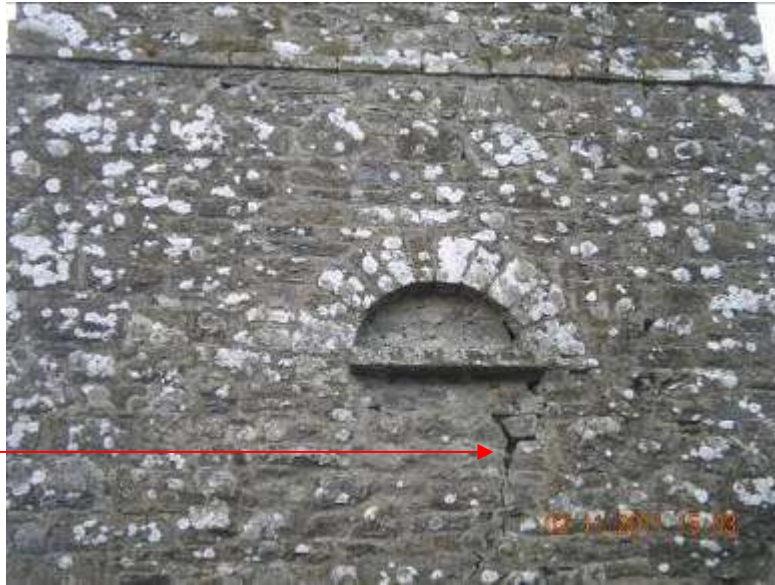
West wall of tower
