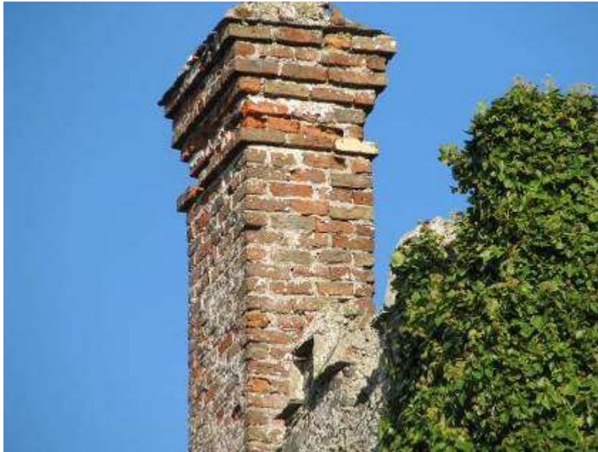
The chimney from the South
