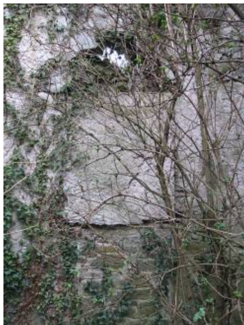
Interior – note lime plaster on north wall
