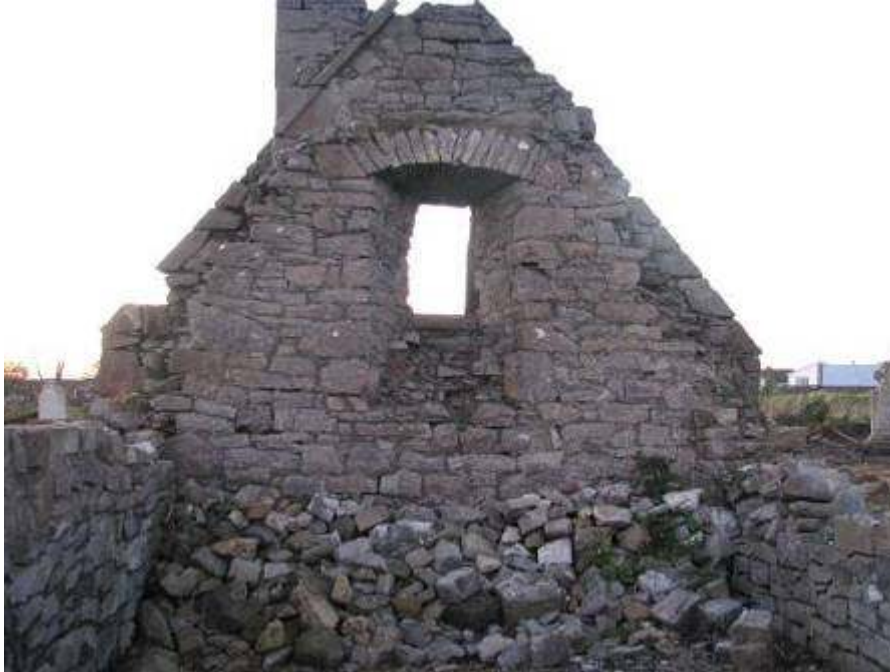
West gable wall, east face
