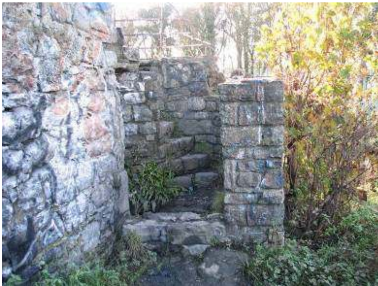
Entrance to spiral stair
