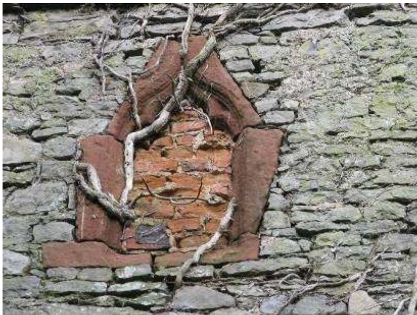
Sandstone Ogee window on south wall
