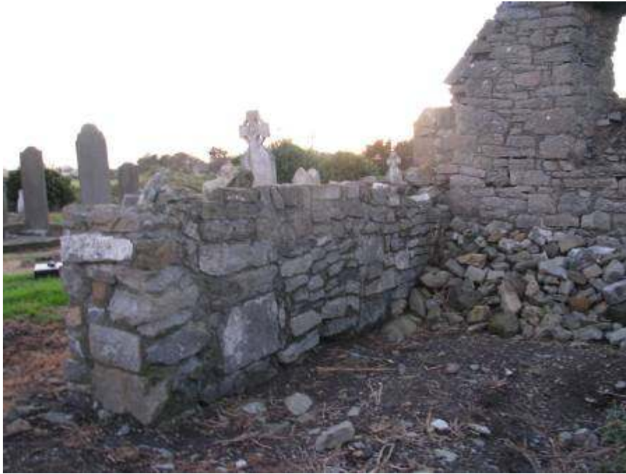
South wall, west end
