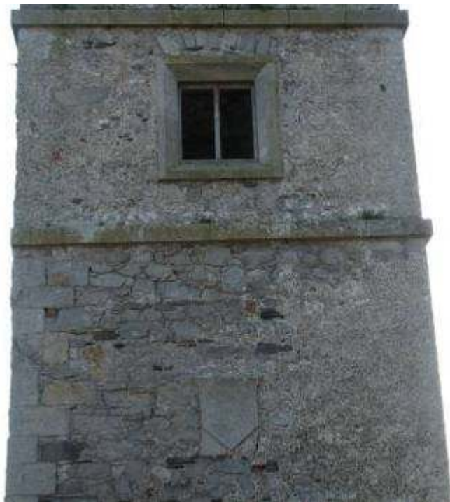
Detail of window frame and wall plaque on north wall
