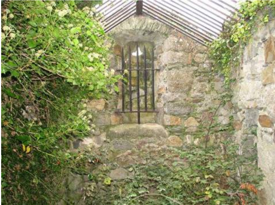
Interior showing the east wall
