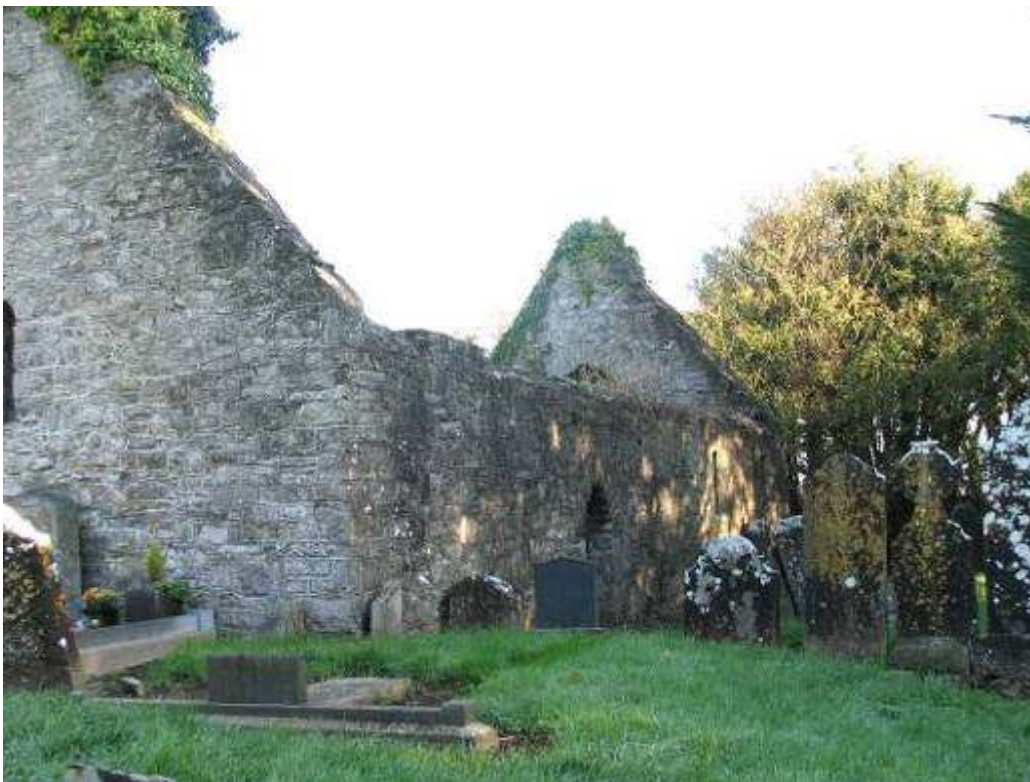
(General view from the south-west)
