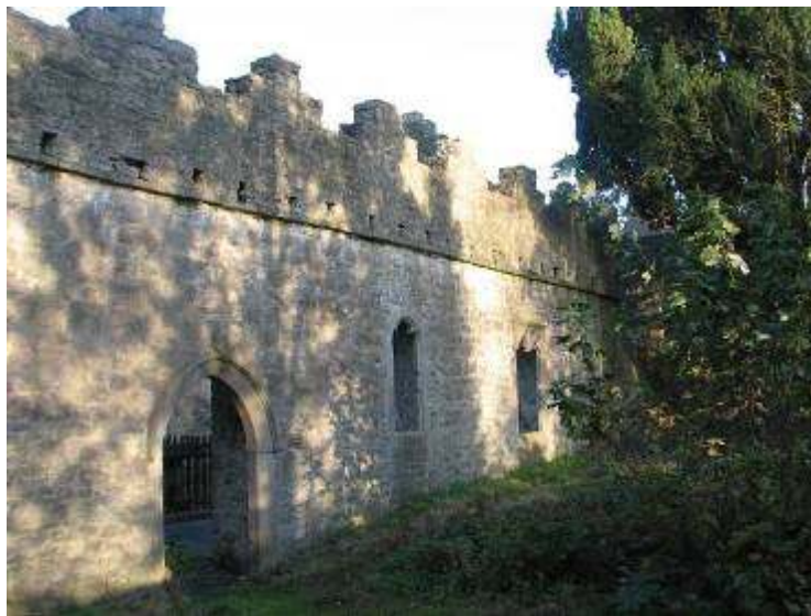
South elevation of nave
