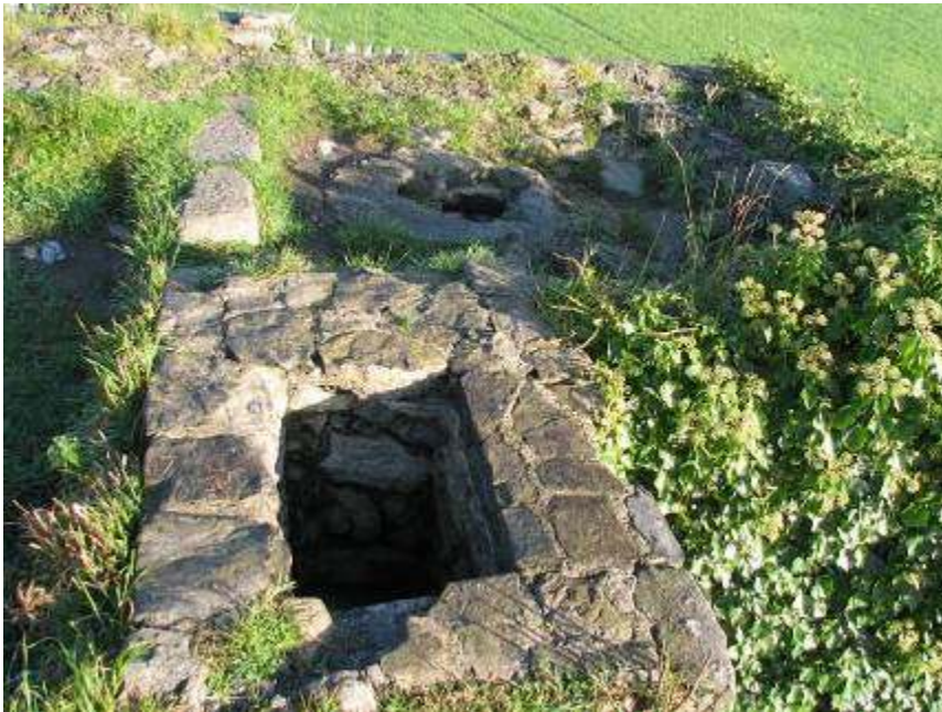
First floor east side – note truncated chimney and north-east tower
