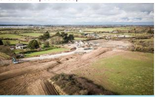
The main activities currently taking place on site include setting out of the alignment and earthworks, excavation for road sub-structures and construction of the road drainage network. One of the most visible elements of the contract will be the earthworks phase and this will take place in the coming months when ground conditions are more favourable.
