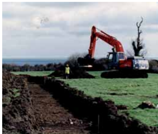
Figure 4: Testing in Bremore
