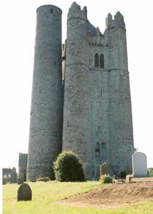
Figure 1: The Round Tower and medieval bell tower at Lusk facing east
