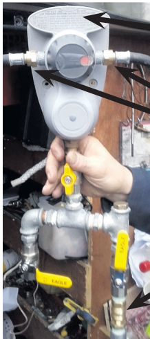
Photograph 9: Low pressure regulator
