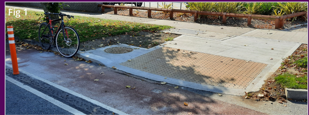
Fig 1. Similar example of road crossing with dished path and tactile paving for improved accessibility, and buff and red coloured protected cycle lanes with bollards.
