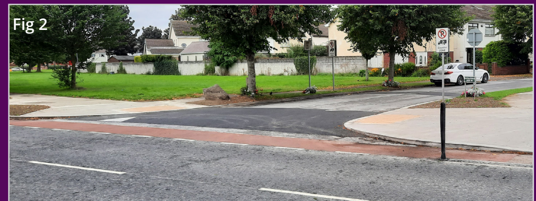
Fig 2. Similar example of extended corners and tactile paving at side roads to make walking safer and slow traffic as it approaches junctions, prioritising people in the community when crossing junctions.
