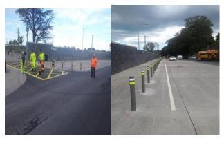
Installation of Bollards on Carrs Lane has commenced with the purpose of a 3m wide pedestrian walkway along the cemetery wall.
