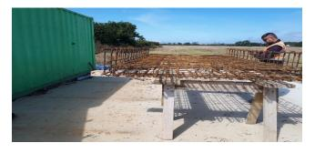
Prefabricating reinforcement for beams and deck
