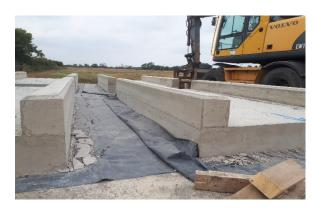
Beams poured and formwork stripped
