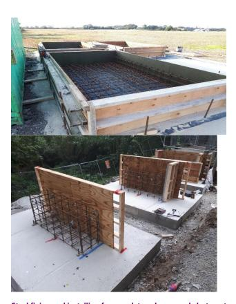
Steel fixing and installing formwork to columns and abutment walls
