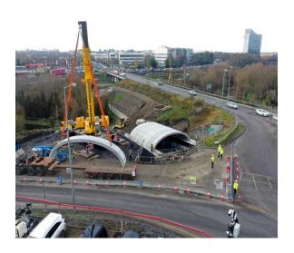
Major bridge construction works were undertaken in December where an arched underpass was installed over the course of two days. Piling works for bridge abutments has been completed this month and retaining walls on adjacent roads are currently being built. Piling works for the central pier will be concluded in January with significant traffic management to be put in place on the N3 from January onwards to facilitate these works.
