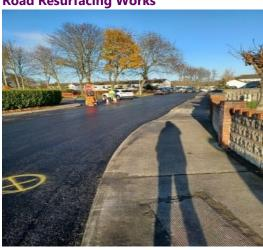
A section of Inbhir Ide Drive was inlaid by a contractor. Millview Rd was also reinstated after Fingal County Council Operations installed road gullies and repaired the surface water lines in December.
