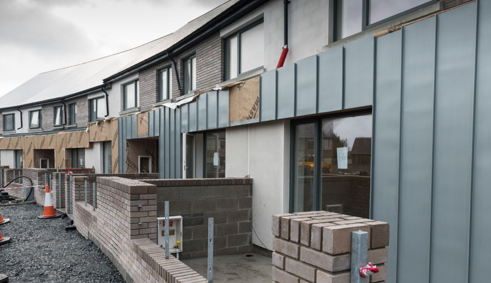
Fingal County Council housing under construction in Racecourse Common in Lusk.
