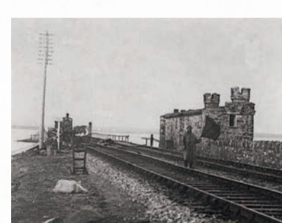
Repairing the viaduct bridge at Malahide after damage caused by the IRA in January 1923 Courtesy of the Malahide Historical Society
