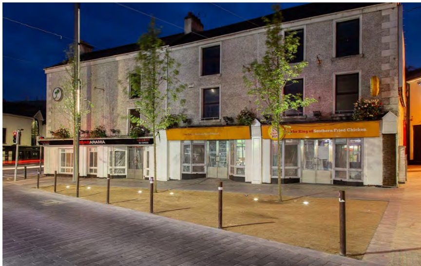
Fig. 9-14: Example of Lighting in the Public Realm
