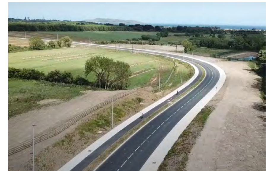
Fig. 1-4: View of Donabate Distributor Road
