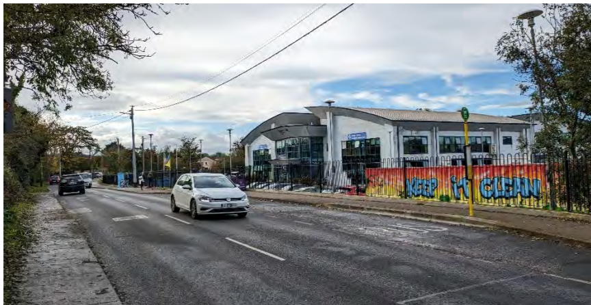
Fig. 6-11: View Northeast along Portrane Road
