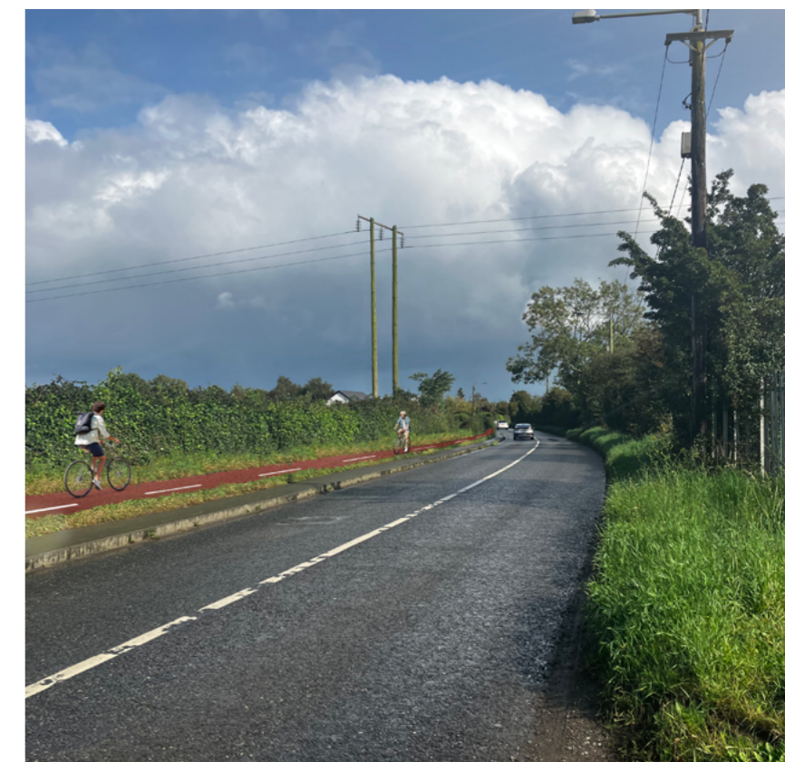
Proposed Cycling infrastructure between Lusk & Rush connecting Lusk to the Train Station.
