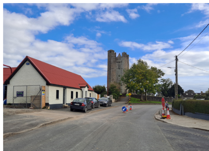
Recently completed Lusk Cultural Centre by the Lusk Community Council beside Lusk Round Tower
