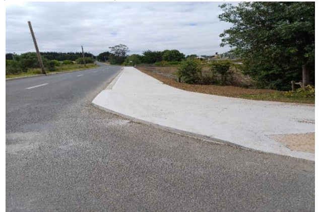
Footpath Works at Kinsealy Lane
