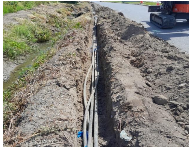
Drainage works at Brooke Lane carried out as part of 2024 Programme of Works. Direct Labour Crews removed all service pipes from the ditch to facilitate dredging works.
