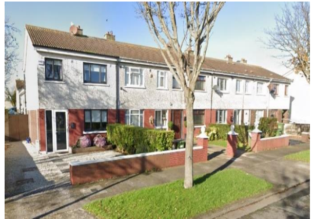
Strandmill - Council and Private Owned Houses - Before
