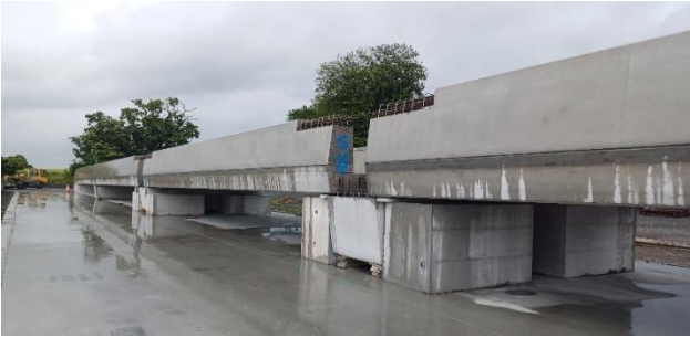
Trial Assembly of spans 7-10 of the bridge - Shay Murtagh Premises
