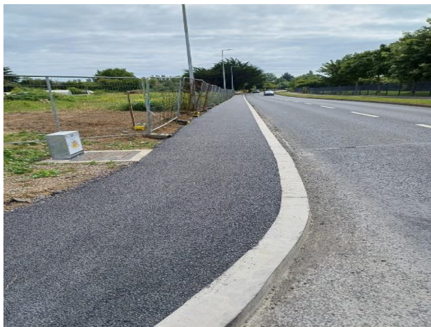
Footpath Works at Malahide Road adjacent to allotments
