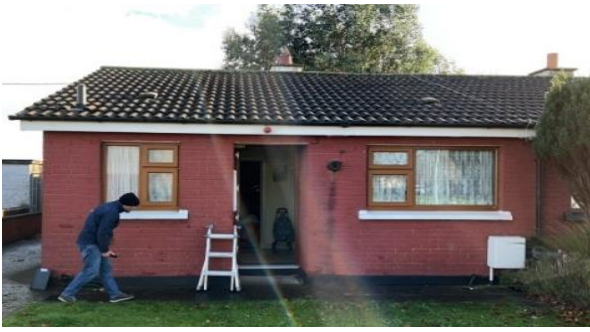
Strandmill Bungalow - Before Retrofit
