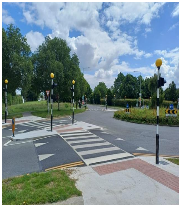
New Zebra crossings at Coolmine Roundabout
