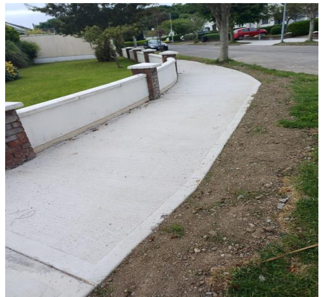
Footpath works in Woodcliffe, Howth
