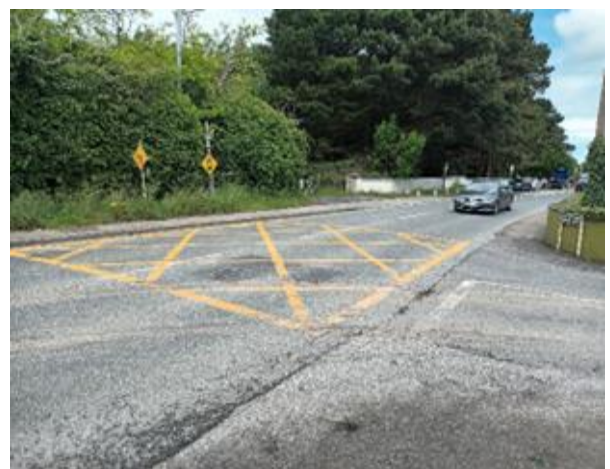
New Yellow Box for junction of Posie Row and Malahide Road
