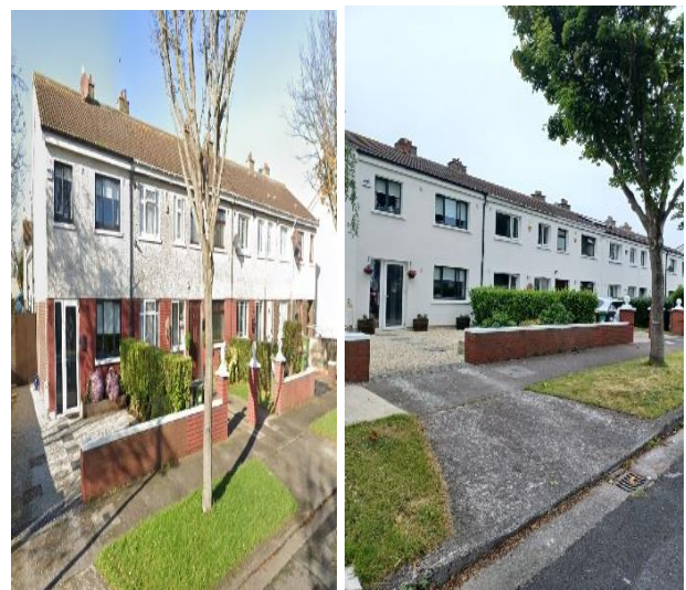
Pre & Post-works – Strandmill Estate, Portmarnock (external wall insulation, new windows and doors, Heat pumps, Attic Insulation and heating controls).
