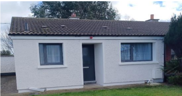
Strandmill Bungalow - After Retrofit
