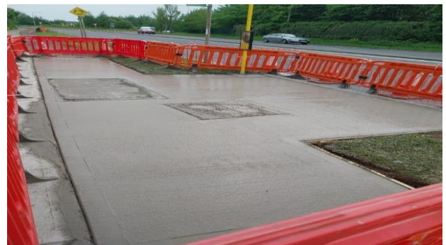
Murrough Road footpath works being carried out by Operations crew.
