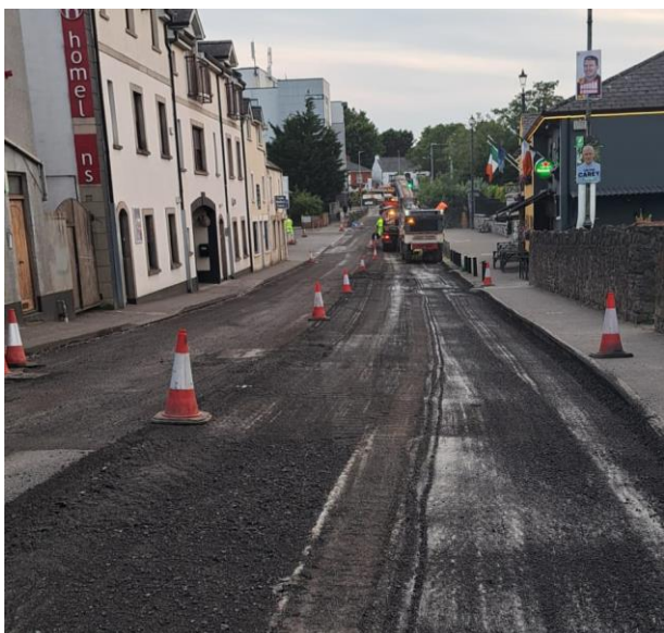
Capital funded resurfacing works on Bridge Street, Swords.
