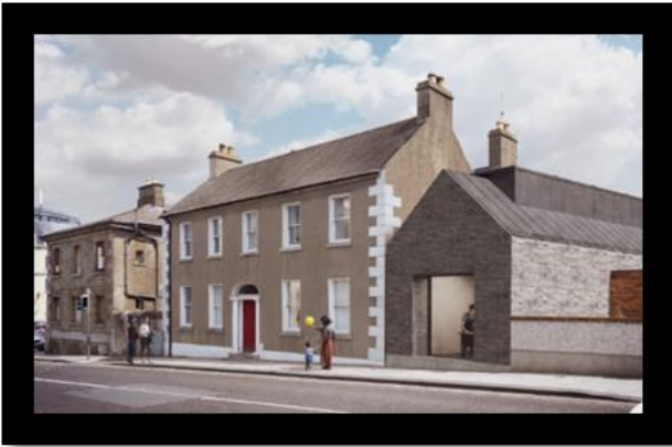
Demolition works on 14 Bridge Street (house known locally as Keelings) have been completed and a temporary Pocket Park has been installed.
