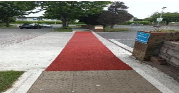
Kinsealy Shopping Centre: New red epoxy resin finish across entrance to highlight pedestrian crossing point.
