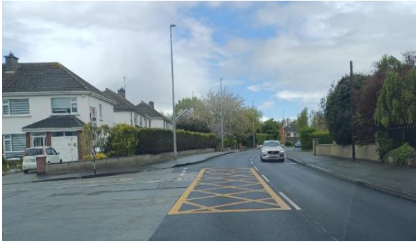
Rathbeale Road – The installation of a yellow box at the junction with Daleview
