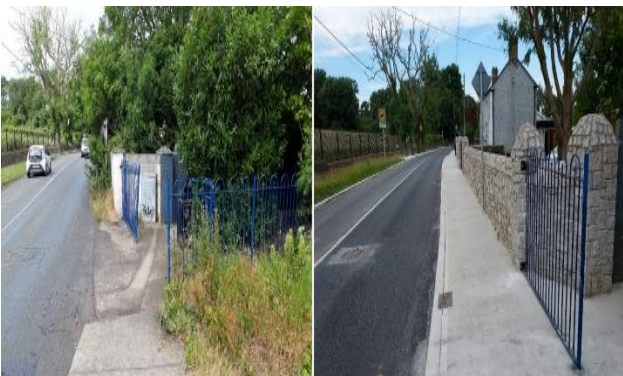
Photographs of Turvey Avenue, pre and post works
