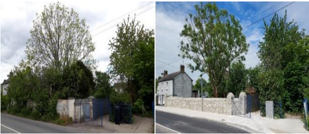
Photographs of Turvey Avenue, pre and post works
