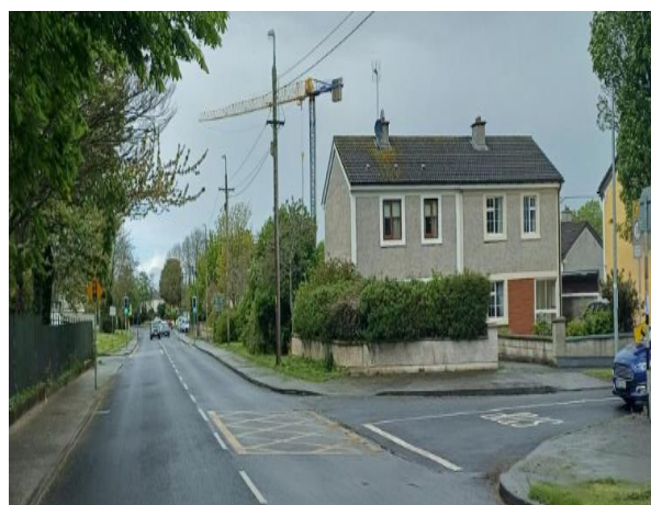
Rathbeale Road – The installation of a yellow box at the junction with Moortown
