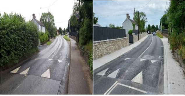
Photographs of Turvey Avenue, pre and post works
