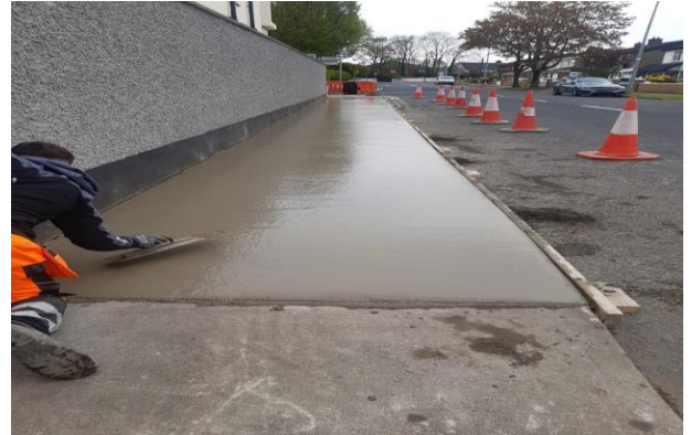
Footpath construction in conjunction with road resurfacing, Roselawn Road
