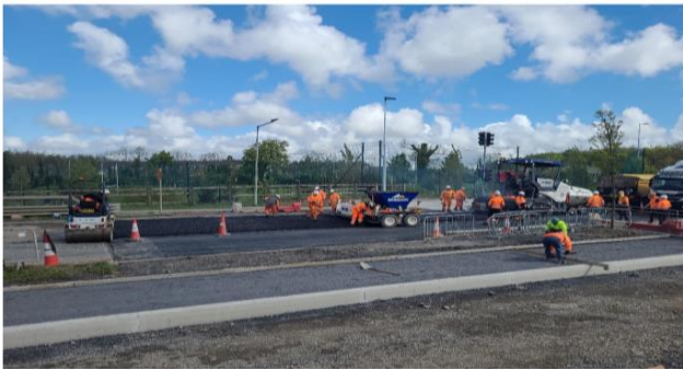
HRA Works - Damastown Roundabout
