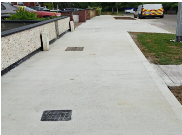
Hilltown Grove, Rivervalley, footpath works carried out by direct labour crew.
