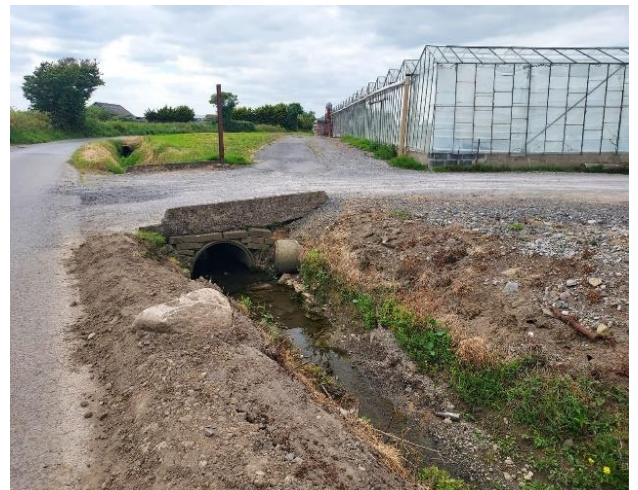
Drainage works at Brooke Lane carried out as part of 2024 Programme of Works. Direct Labour Crews removed all service pipes from the ditch to facilitate dredging works.
