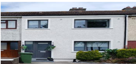
Strandmill - After Retrofit
