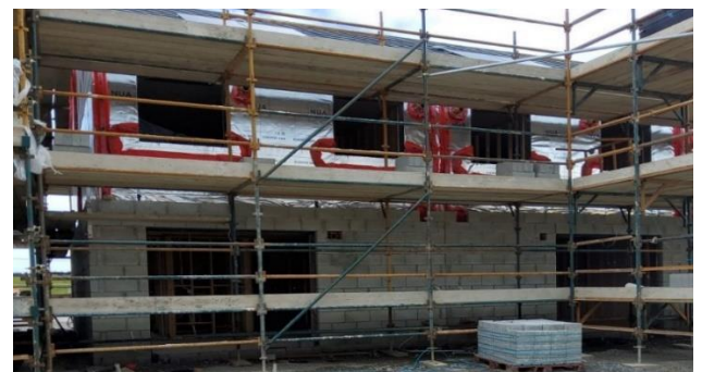
Checking fire stopping in a building in Donabate.
