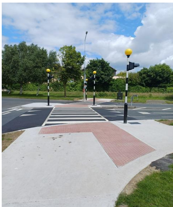
New Zebra crossings at Coolmine Roundabout
