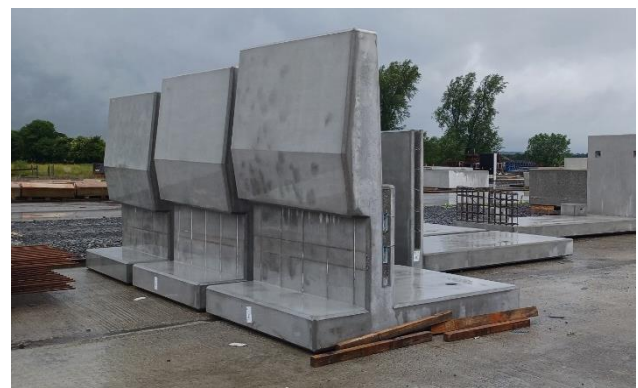
Precast units for the southern ramp – Shay Murtagh Premises
