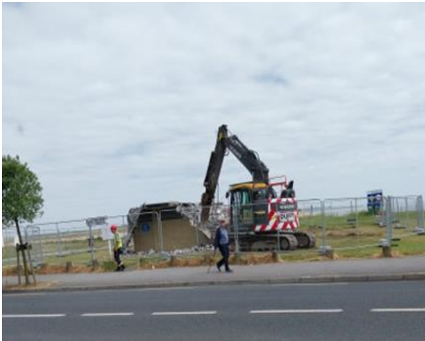
Demolition works on Malahide Beach toilets have commenced.
