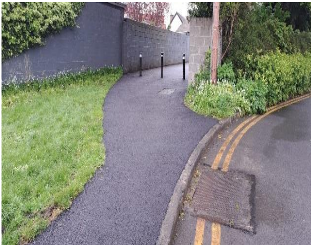
Seatown Lane; resurfacing works as part of the Revenue funded Programme of Works.
