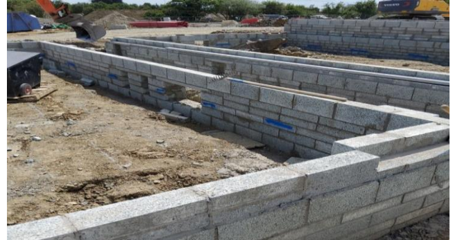
Checking rising walls in a housing development in Balbriggan
