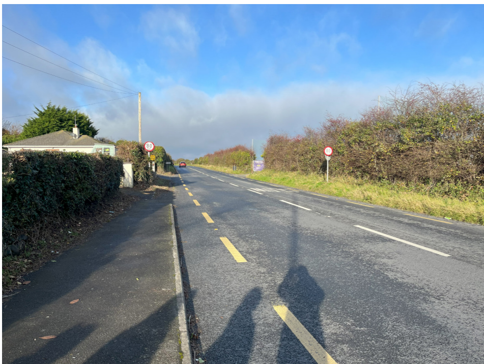
Figure 6.4: Footpath on R132 Route finishes just north of Bremore Cottages junction
