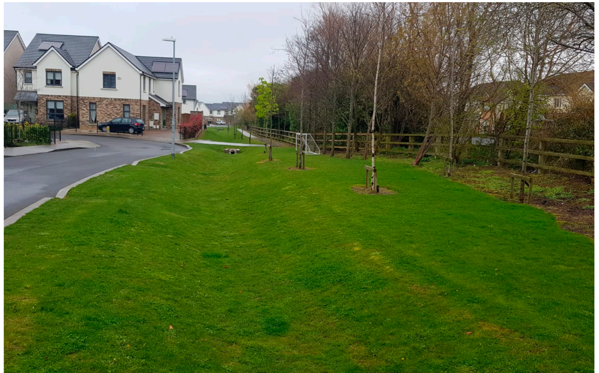
Figure 7.2: Sustainable drainage swale at The Green residential development, Oldtown, Swords
