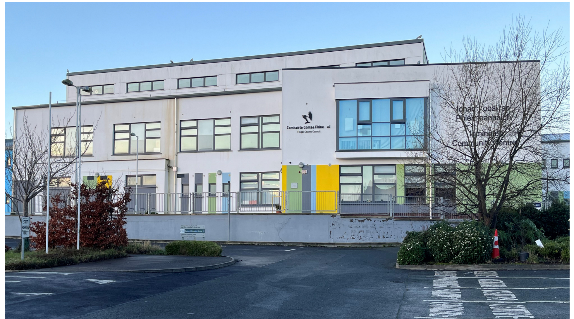
Figure 8.1: Flemington Community Centre
