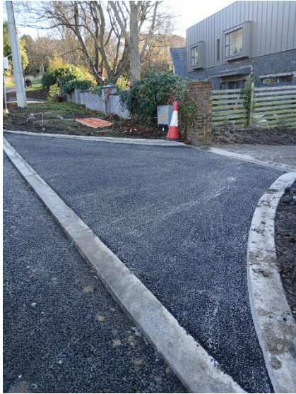
Tarmac works complete
