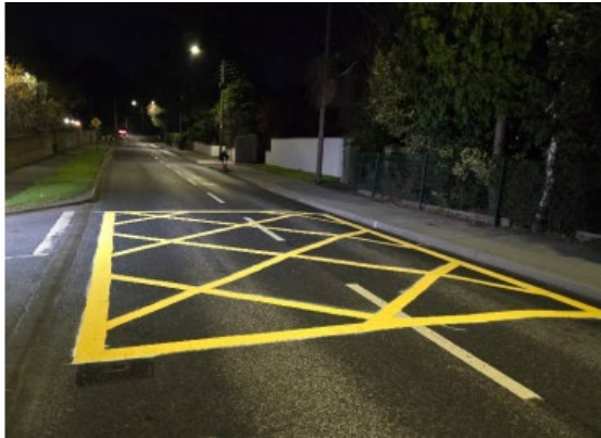
Swords – R106 Malahide Road- Yellow Box markings to aid traffic flow at Mountgorry Wood
