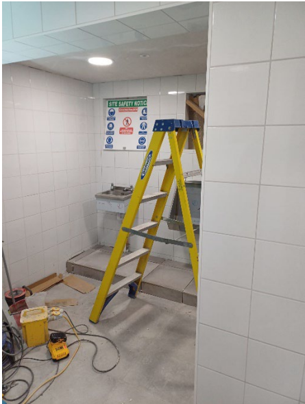
Works underway at the Portmarnock Beach toilets.
