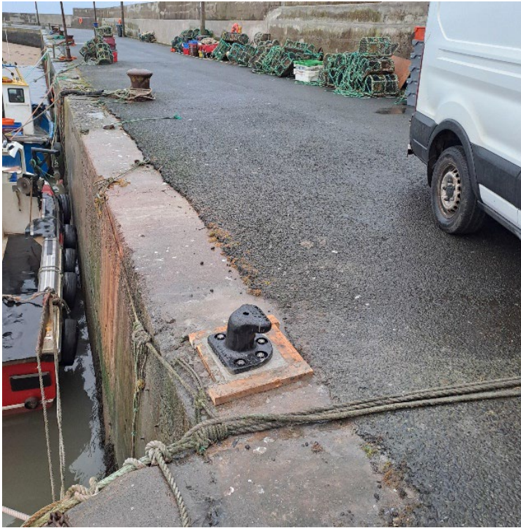
Installation of 5 new mooring bollards along the pier at Loughshinny Harbour.
