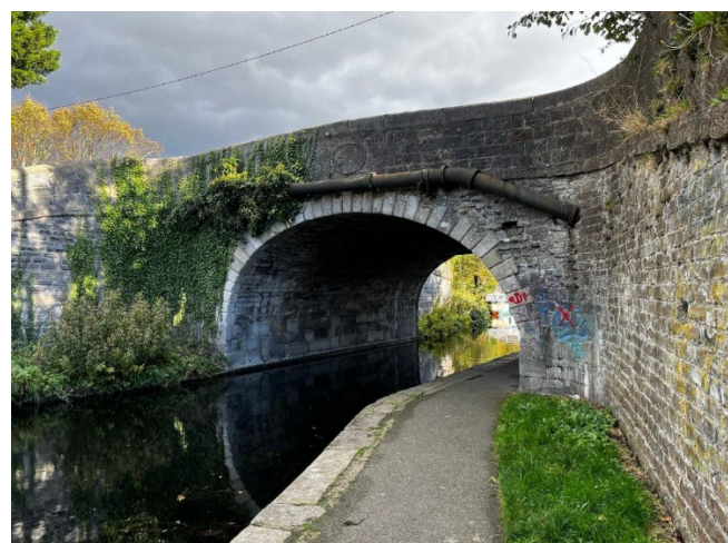
View of the Granard Bridge and the existing underpass
