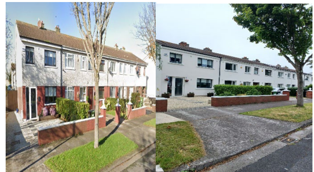
Pre & Post-works – Strandmill Estate, Portmarnock (external wall insulation, new windows and doors, Heat pumps, Attic Insulation and heating controls).
