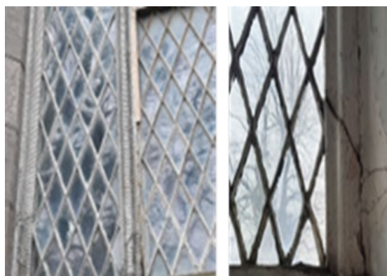
HSF - Before Repairs to Window Timber Tracery
