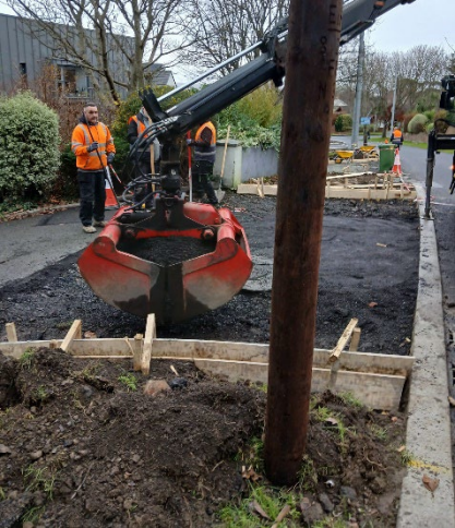
Prior to replacement of kerbs & tarmac
