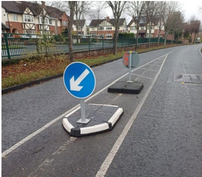
Newly installed modular island on Diswellstown Road
