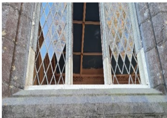
HSF - Repaired Window Tracery – St Columbas Church, Swords
