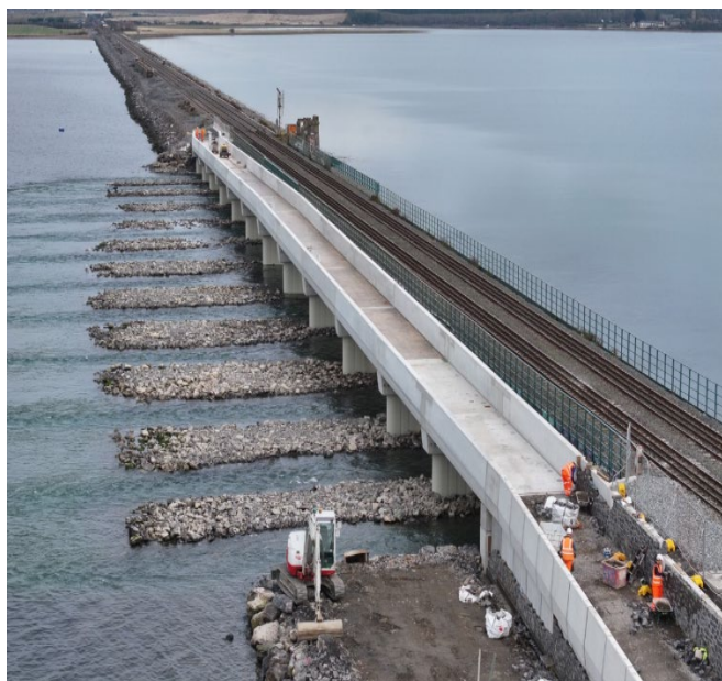
New estuary bridge and ramps looking northwards towards Donabate
