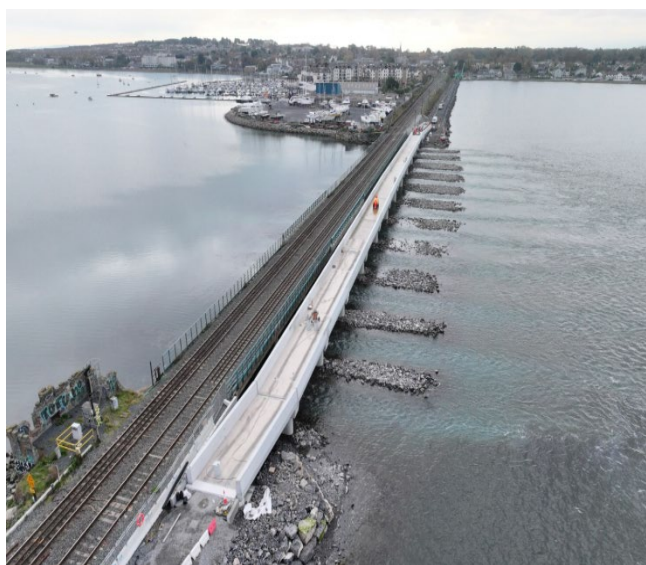
New estuary bridge and ramps looking southwards towards Malahide.
