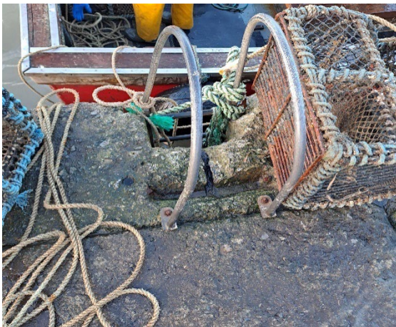
The embarkation ladder at Loughshinny Pier has been repaired and widened to allow safe access and regress.
