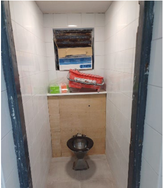
Works underway at the Portmarnock Beach toilets.
