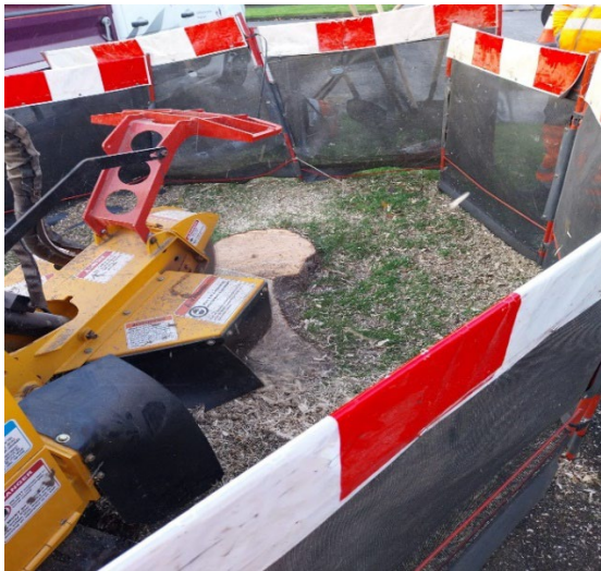
Tree stump removal been carried out in Delwood Lawn
