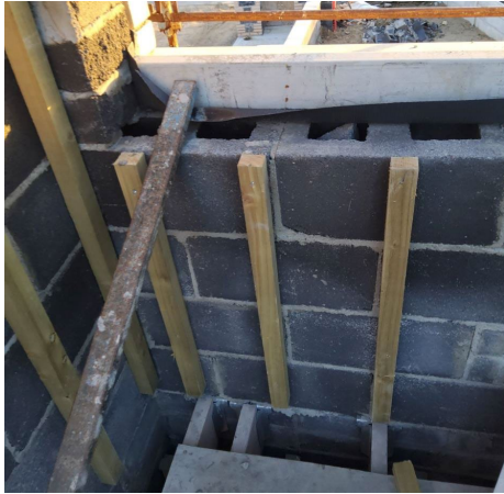
Checking window detail in a house in Rush.
