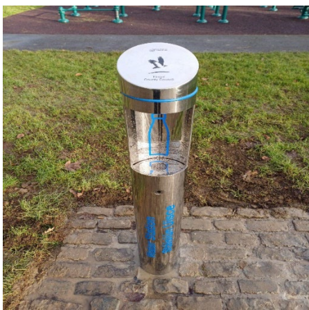
New water fountains installed at Hartsown Park Dog run recently
