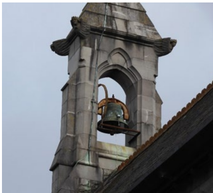
BHIS - Repaired Belltower and Roof - St Mochtas Church, Castleknock
