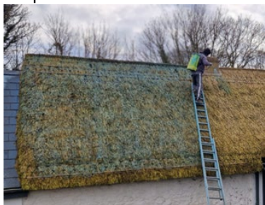
AHF Project - 'Bluestone' treatment to prevent rot and extend life of thatch - Balscadden, Balbriggan
