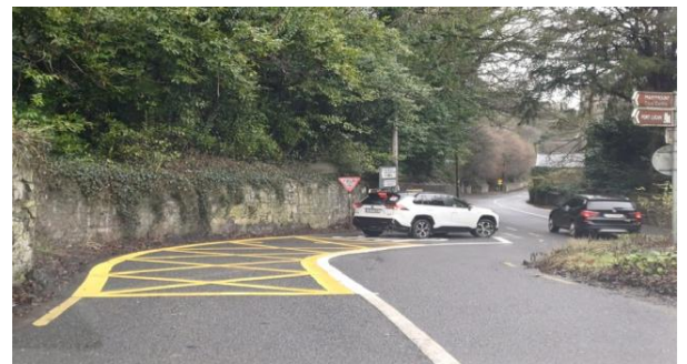
Yellow box and STOP markings repainted at the bottom of Tinkers Hill.
