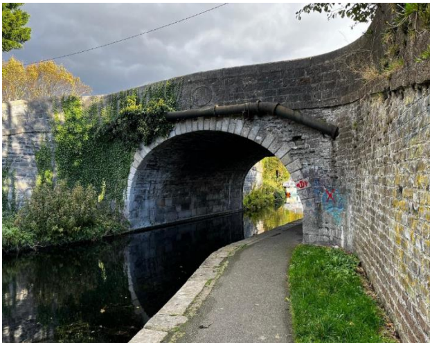
View of the Granard Bridge and the existing underpass
