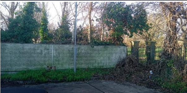
Planting Works carried out in Luttrell Park Court as part of Programme of Works.
