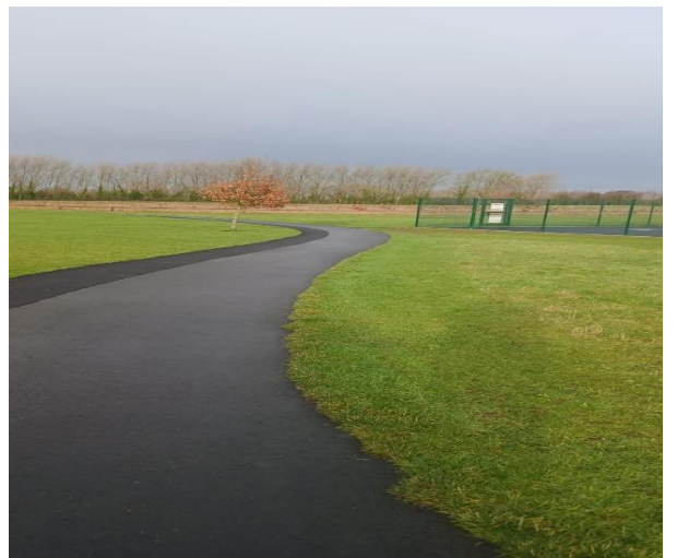
Footpath Widening St Catherine's Park
