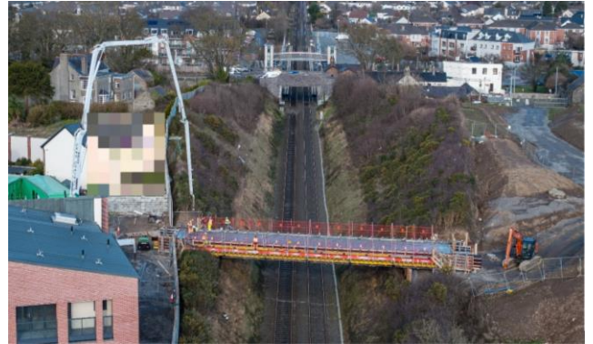
Image of the bridge over the railway (looking towards Donabate)
