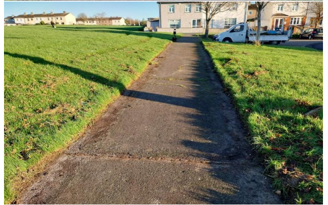
Edging works been carried out at Corduff Green
