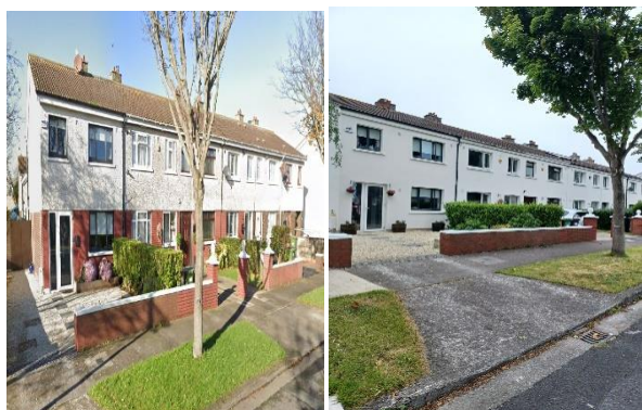
Pre & Post-works – Strandmill Estate, Portmarnock (external wall insulation, new windows and doors, Heat pumps, Attic Insulation and heating controls).
