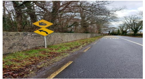
New SLOW Road marking and yellow rumble strips added to Tinkers Hill.
