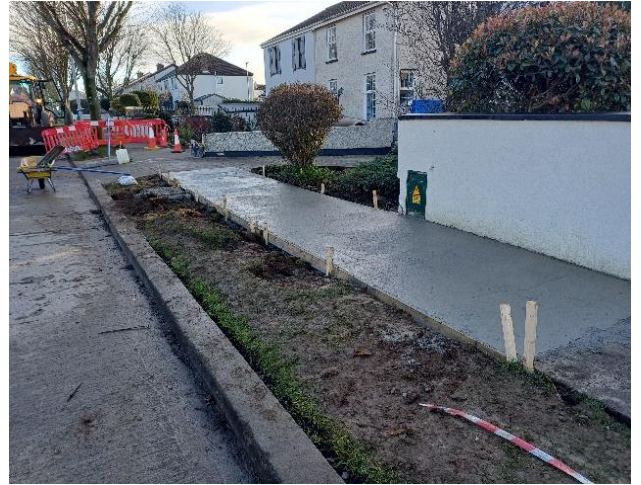
Roads crew replaced storm damaged footpath at Limetree Avenue Portmarnock
