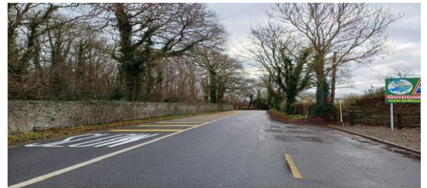
New SLOW Road marking and yellow rumble strips added to Tinkers Hill.
