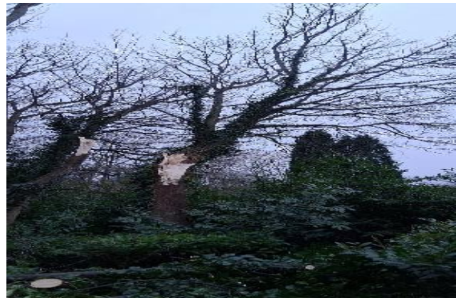
Tree damage on Mc Alister's gate, Crew dealt with limb on the ground and tree surgeon brought in to make safe the remainder of the standing tree
