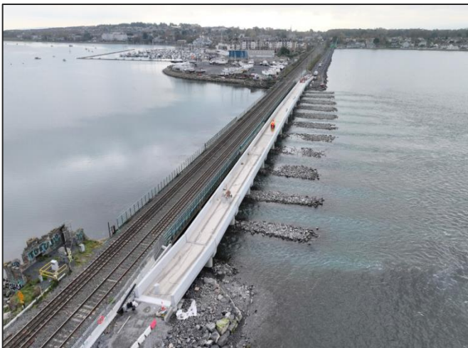
New estuary bridge and ramps looking southwards towards Malahide
