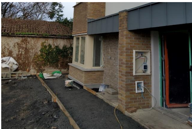
Checking level access to a house being built in Castleknock
