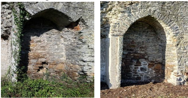
Figs9&10 Before and After repair of arch and buttress
