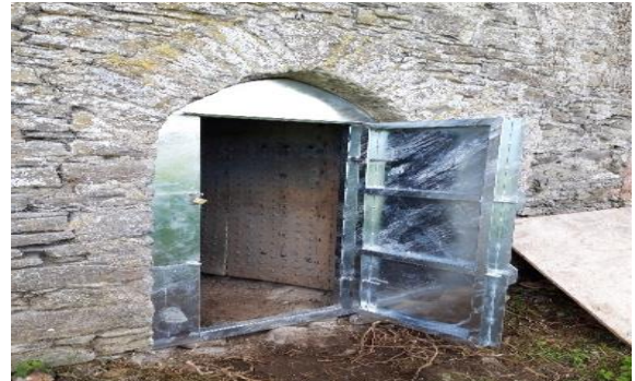
Fig5 Access Door protecting a studded 17/18 th century door
