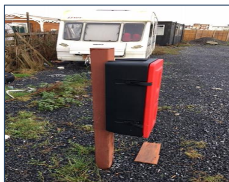
Example of a standalone fire extinguisher pole
