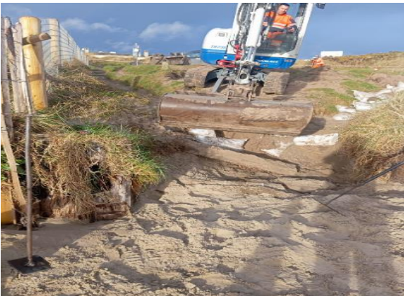
Access to Portmarnock Beach-Before works carried out
