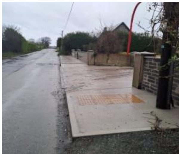
Installation of new footpath along Kinsealy Lane.
