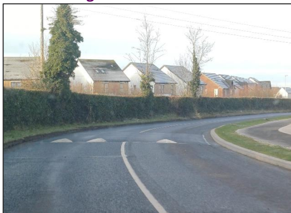
Repainted shark teeth on the Hollywoodrath Road.
