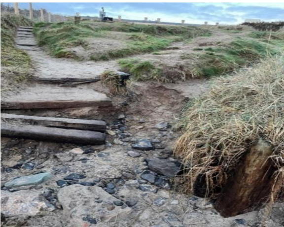
Damage at Portmarnock Beach walkway.
