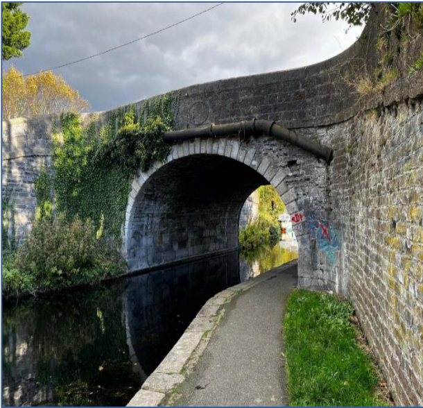
View of the Granard Bridge and the existing underpass
