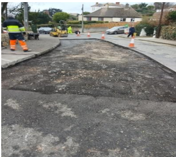
Road patching in St. Laurence's Howth
