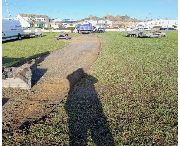
Upgrading of paths Portmarnock
