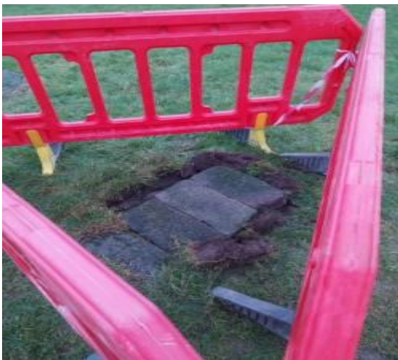
Manhole repairs and manhole replacement in Porterstown Park at the clubhouse.
