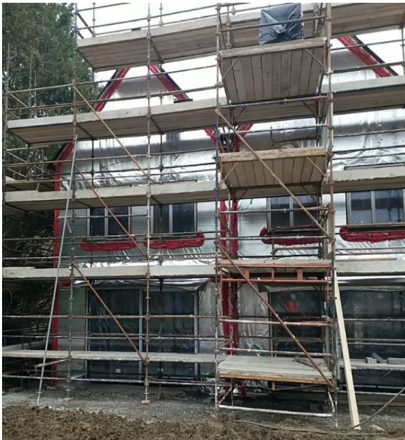
Checking insulation and fire stopping on a house in Malahide
