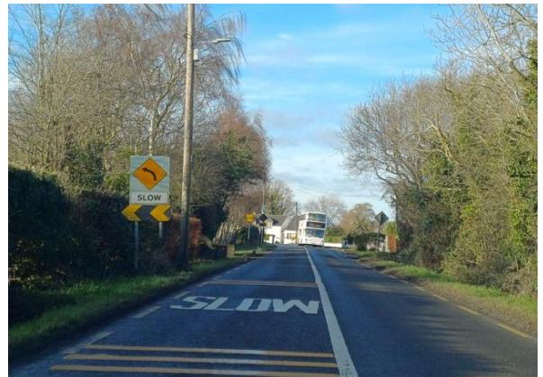
SLOW markings associated yellow rumble strips repainted on Westmanstown Road.
