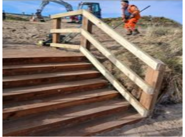
Access to Portmarnock Beach-After works carried out
