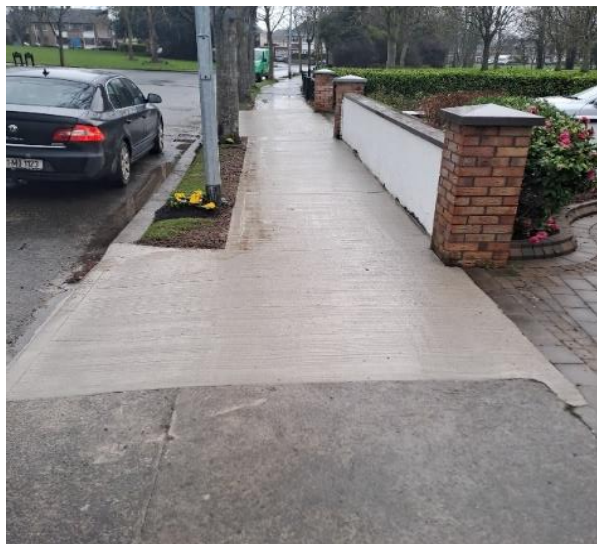
Footpath bay replacement in Ardilaun Estate, Portmarnock.
