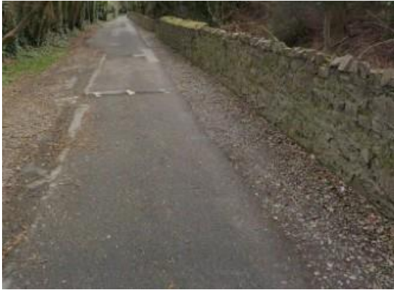
Before & after photos of road overlay at Black Avenue Road St Catherines Park, overlay upgrade of 270m as well as drainage works carried out.
