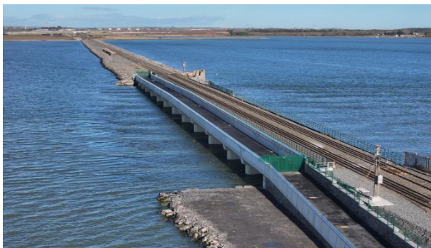
New estuary bridge and ramps looking northwards towards Donabate
