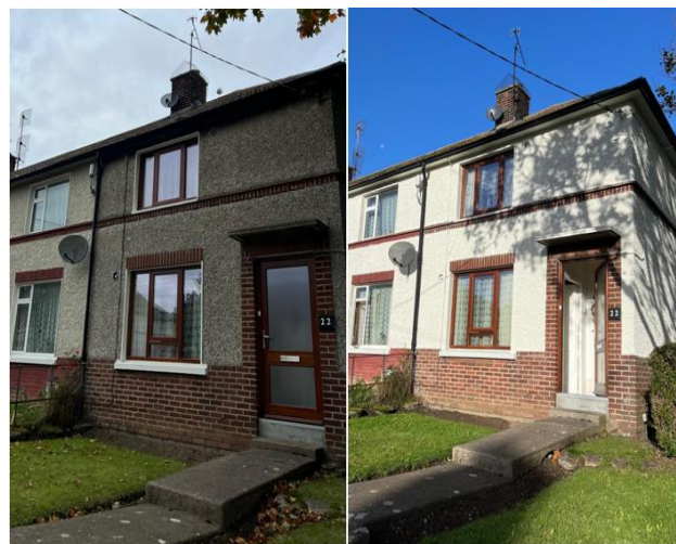
Scheme Painting Before (L) & after (R) Grace O'Malley Estate
