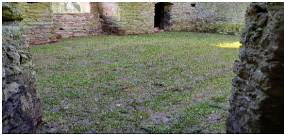
Fig8 After - Puddling clay and layer grassy sod installed
