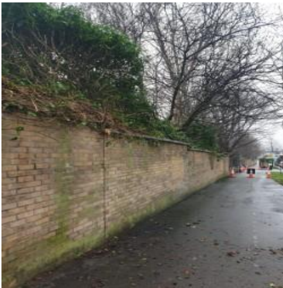
Footpath cleaning Snugborough Road
