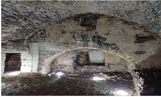
Fig7 After - lintel on left replaced and vaults repaired
