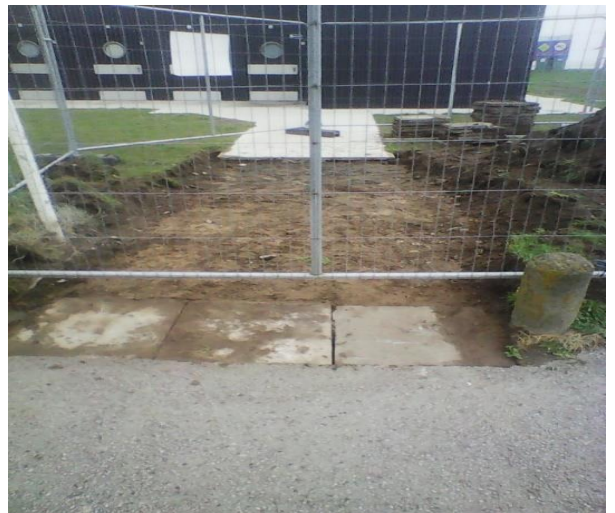
Exterior snag works commenced at Malahide Howth new toilet units
