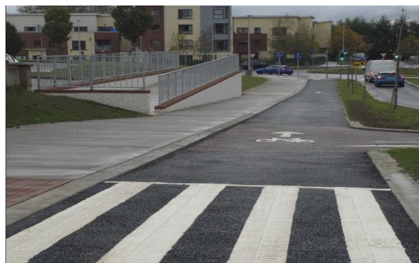
Southbound segregated cycle track and new ramp on Wellview Road
