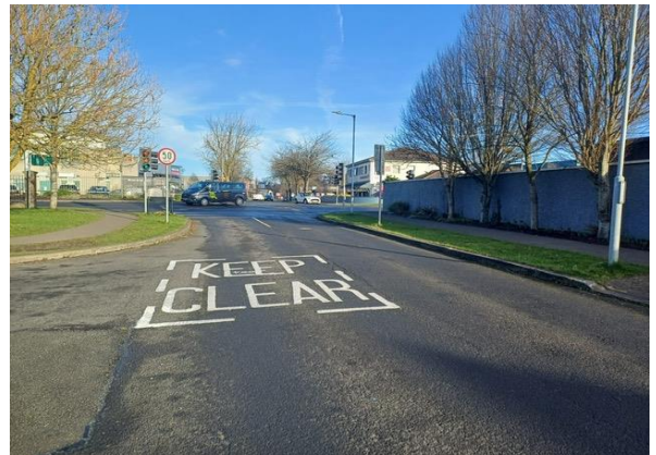
KEEP CLEAR road marking applied to the junction of St. Mochtas Road and St. Mochtas Park
