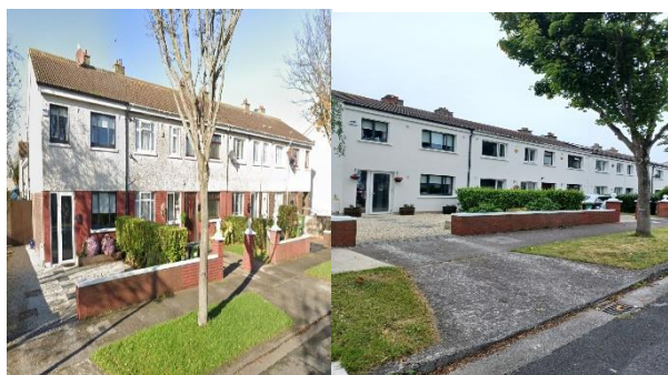
Pre & Post-works – Strandmill Estate, Portmarnock (external wall insulation, new windows and doors, Heat pumps, Attic Insulation and heating controls.
