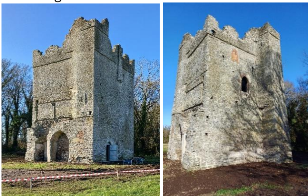
Figs1&2 Lanistown Castle -East and north facades after the works
