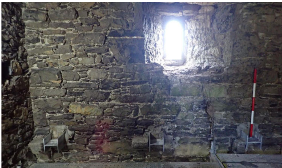
Plate 27: H-brackets positioned beside the corbels, east wall.
