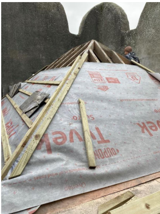
Plates 32-33: Slates removed.
