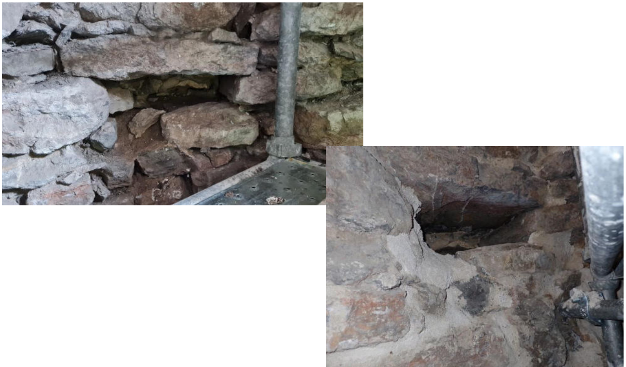
Plate 11: Beam hole 3 before and after re-pointing
