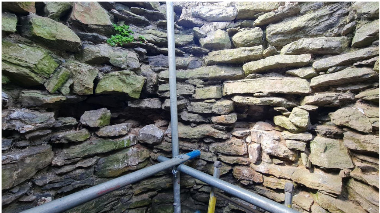
Plate 17: Beam holes 2 (left) and 1 (right) before re-pointing. The distance between them is 1.50m centre to centre, but the wide-angle view distorts this somewhat.
