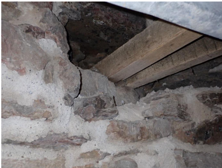
Plate 13: Beam hole 4 after re-pointing but with the wooden beams still in position
