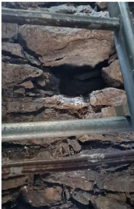
Plate 14: Beam hole 1 before and after re-pointing
