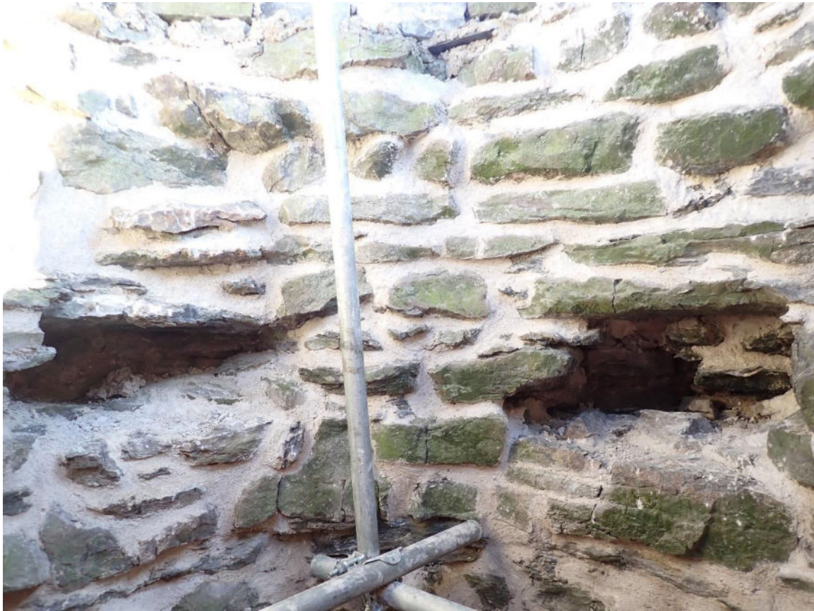
Plate 20: Beam holes 4 and 3 after re-pointing.
