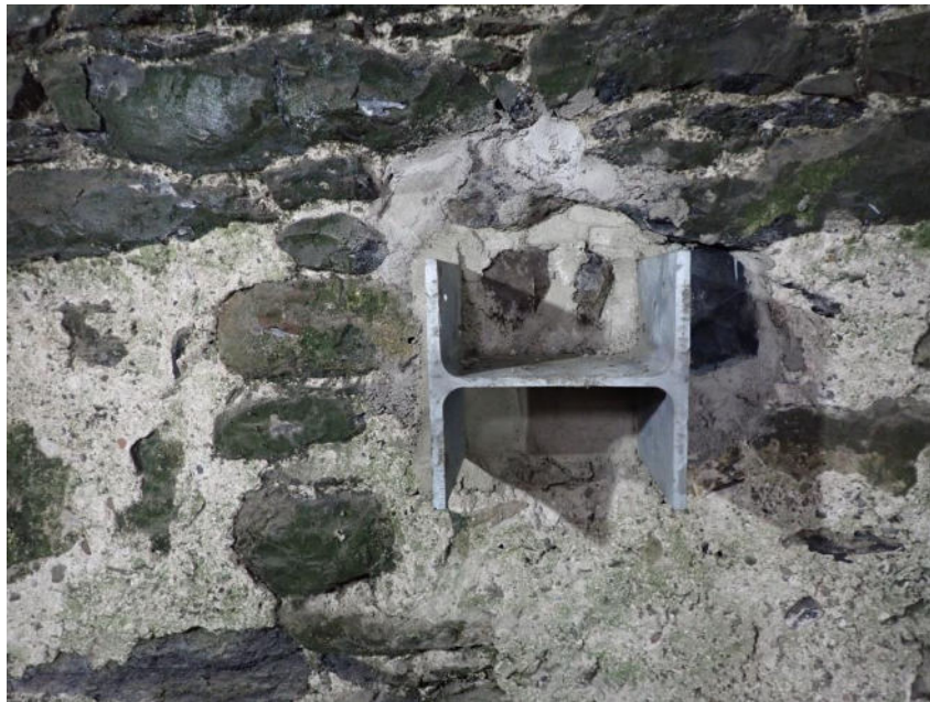
Plate 26: Stone replacing the brick infilling of the holes around the brackets.
