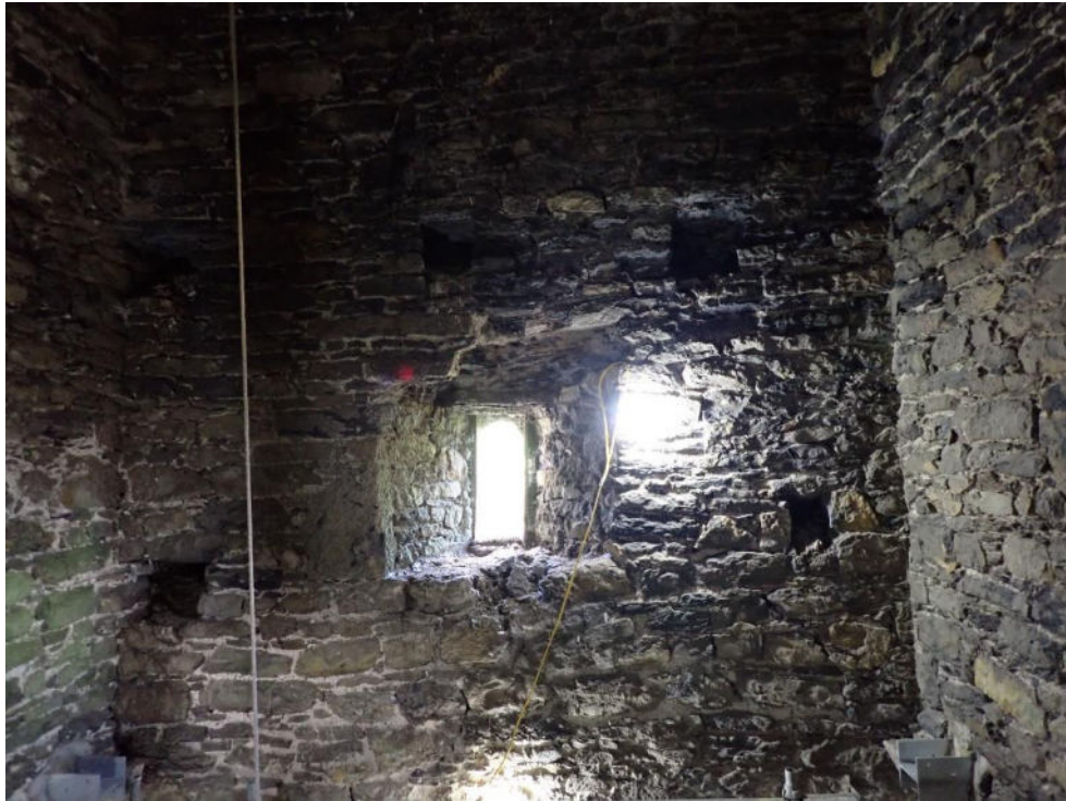
Plate 37: View of the north wall with joist sockets above the window level, below the bell floor. Note the possible putlog holes lower down.
