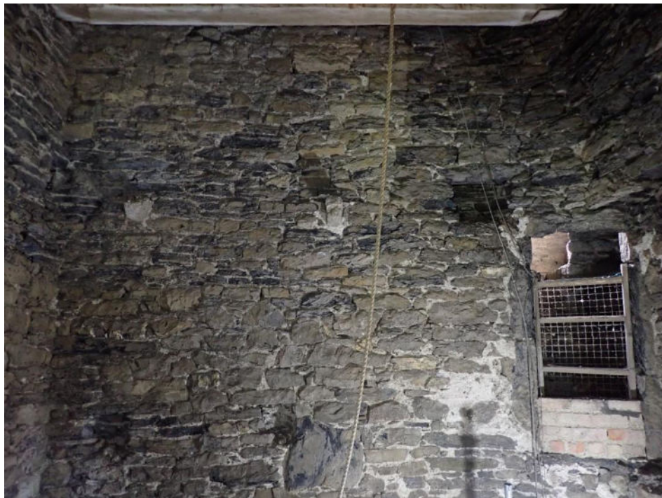
Plate 36: View of south wall with two corbels and one socket below the bell floor level
