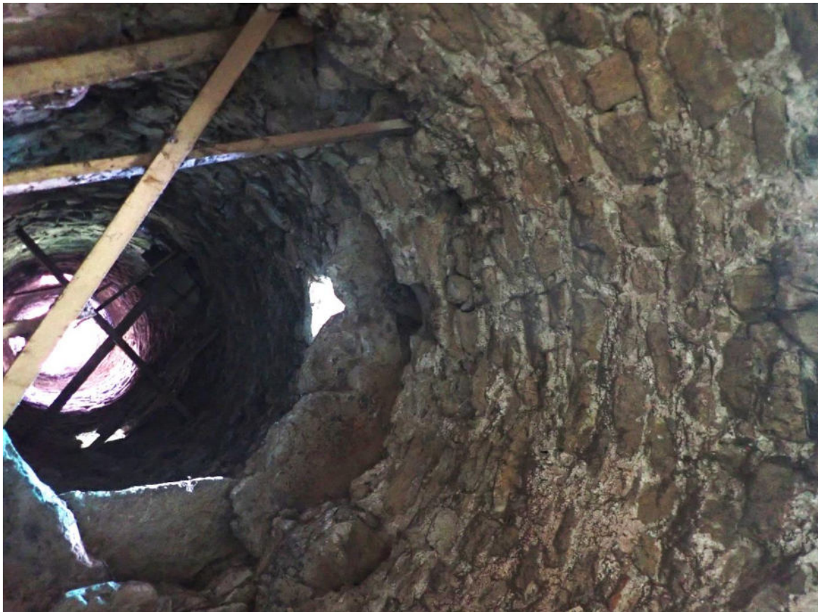
Plate 2: Looking up towards underside of corbelled stones which have protected the mortar from weathering. Taken in 2023 before the beams were removed.
