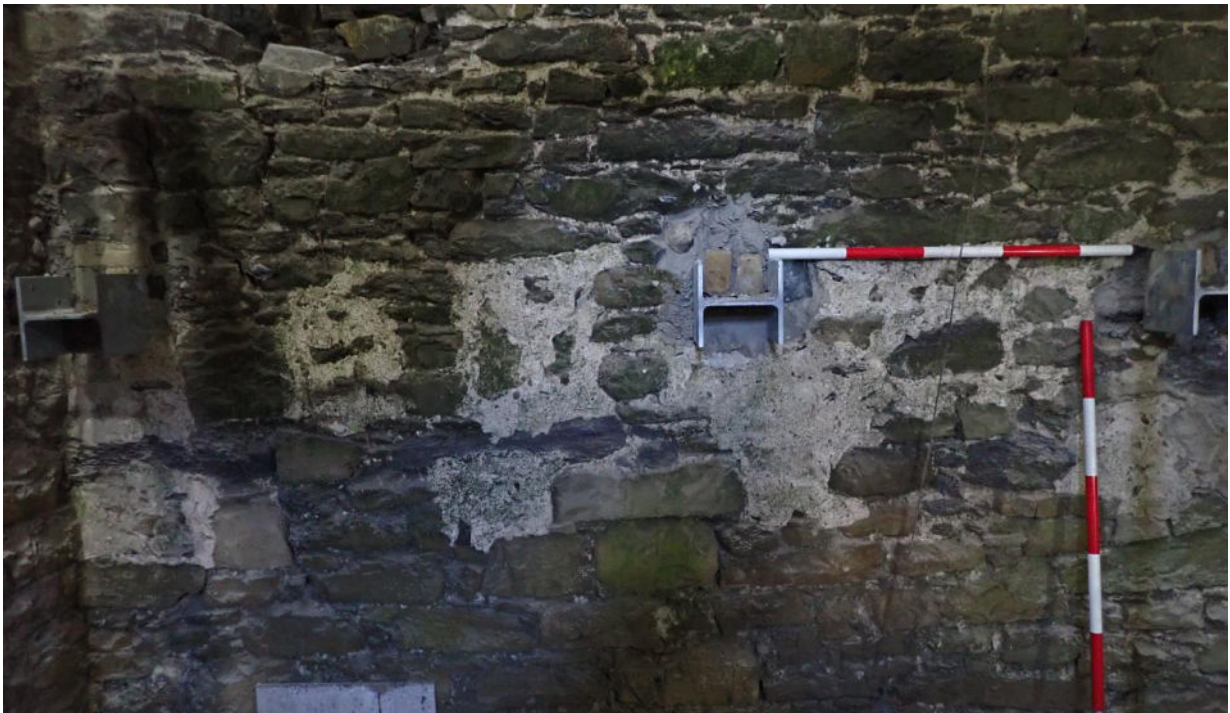
Plate 22: First floor east wall with H-brackets inserted from the NE (left side) corner to centre. Note the lintel-like stones in the centre and above the horizontal ranging rod
