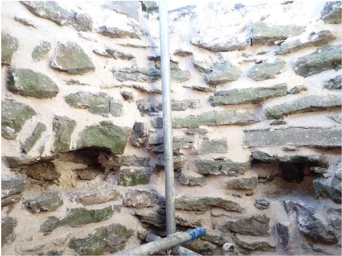
Plate 18: The same beam holes, 2 and 1, after re-pointing.
