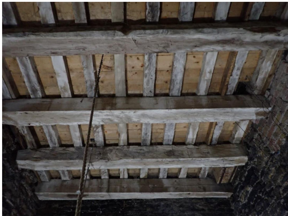
Plate 38: Underside of bell floor with east wall showing brick infill
