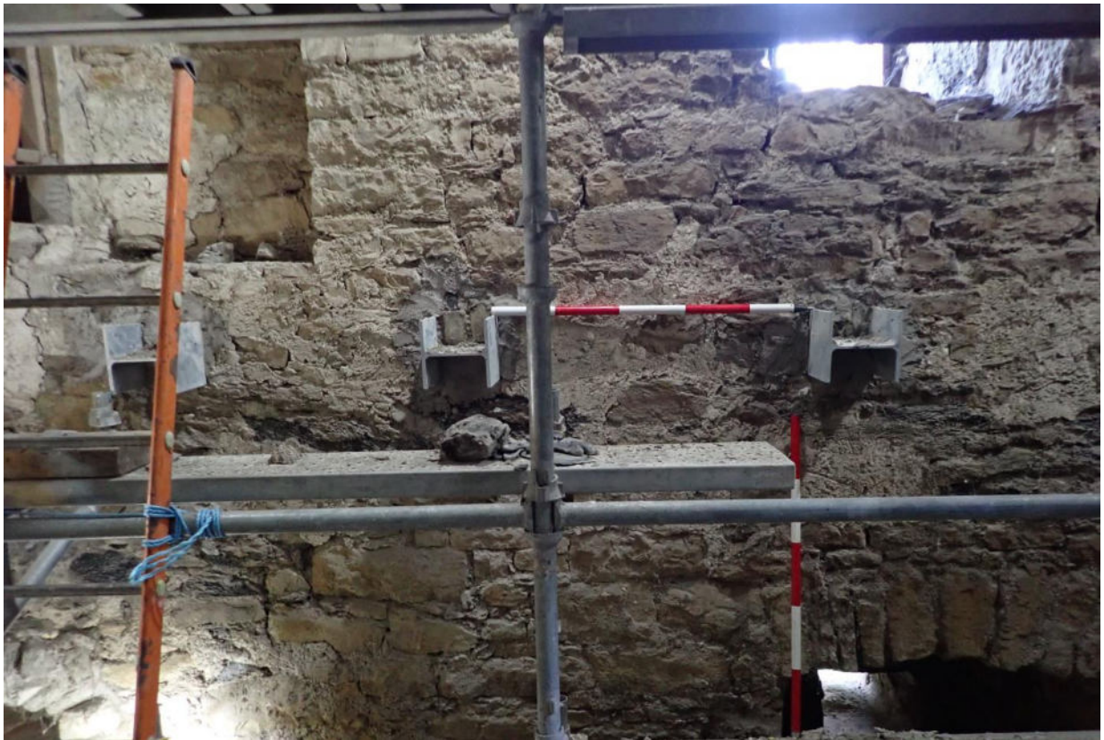
Plate 24: Second floor, west wall, brackets from SW corner at the door to the centre.
