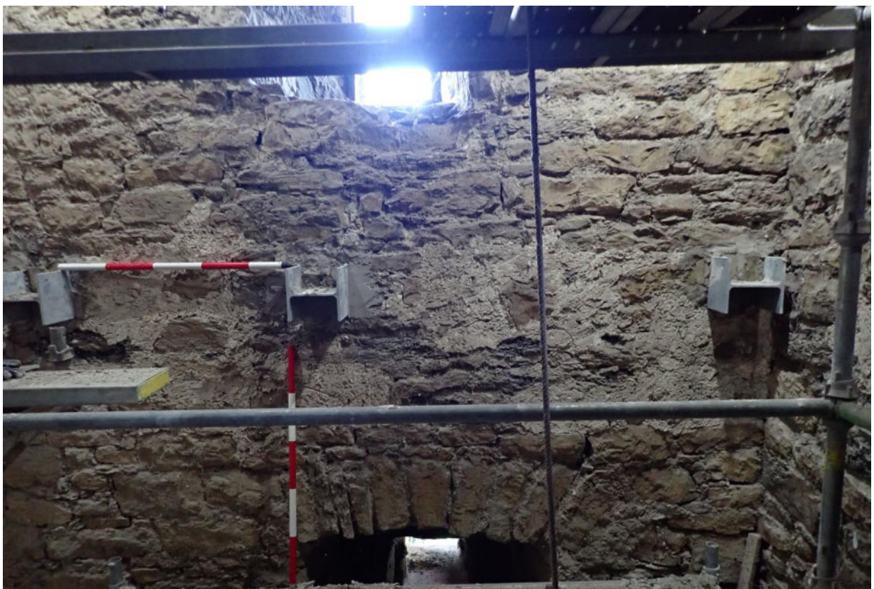
Plate 25: Second floor, west Wall, brackets from the centre to the NW corner.
