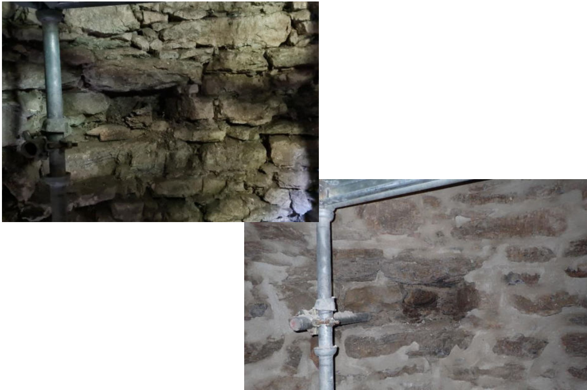
Plate 8: Beam hole 4 before and after re-pointing.
