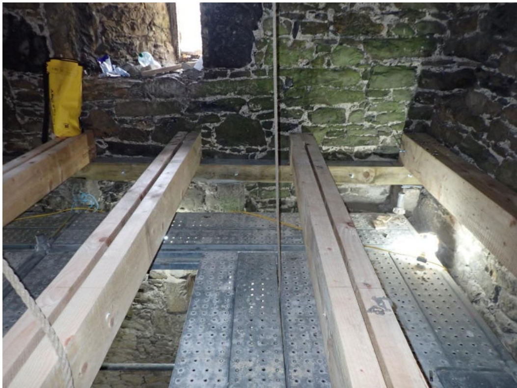
Plate 29: Beam over the corbels, east wall, with joists above.
