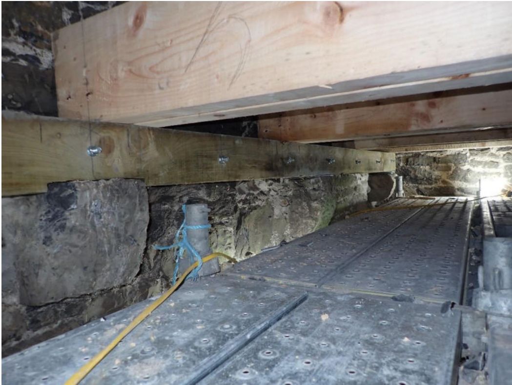
Plate 28: Detail of beam on corbels, west wall, with floor joists above.
