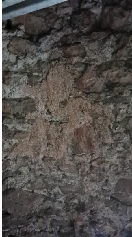
Plate 1: Wall in Floor 1, entrance, retaining pointing and possible plaster of unknown date
